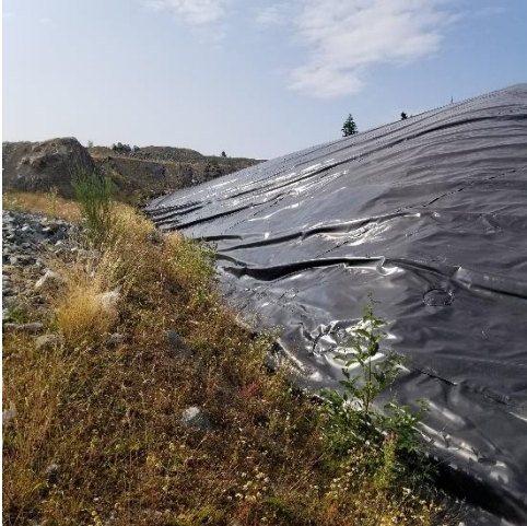
PEA – liner near NE corner
