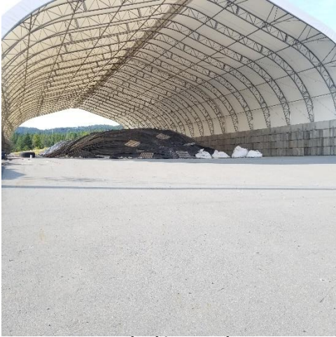
SMA - looking south
