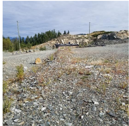
Leak and leachate detection works
