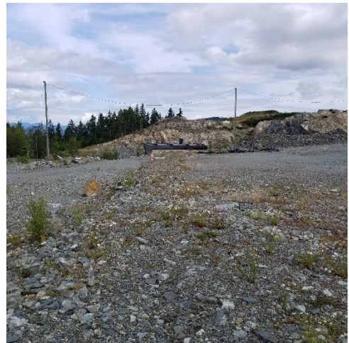
Leak and leachate detection works
