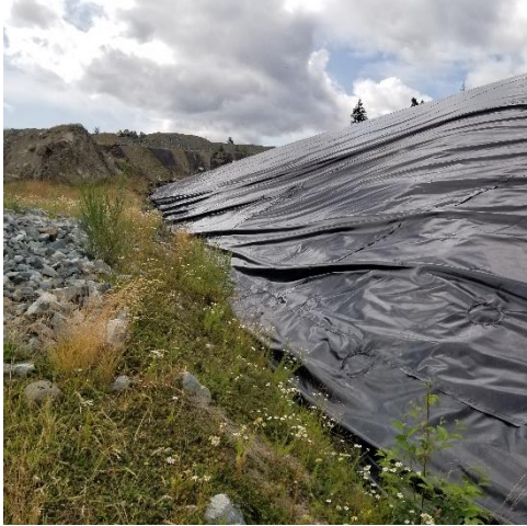
PEA – liner near NE corner
