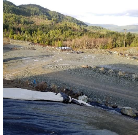
Site – Looking Northwest
