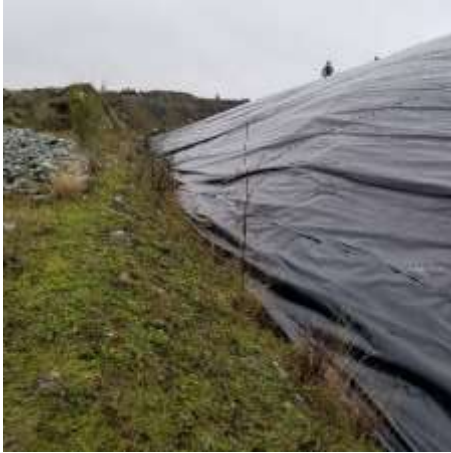
PEA – liner near NE corner
