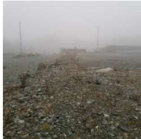
Leak and leachate detection works
