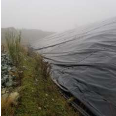
PEA – liner near NE corner
