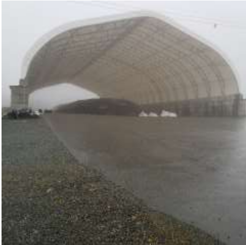
SMA - looking south
