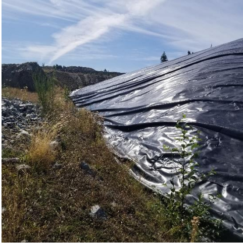
PEA – liner near NE corner
