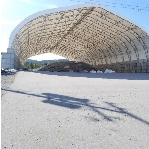
SMA - looking south
