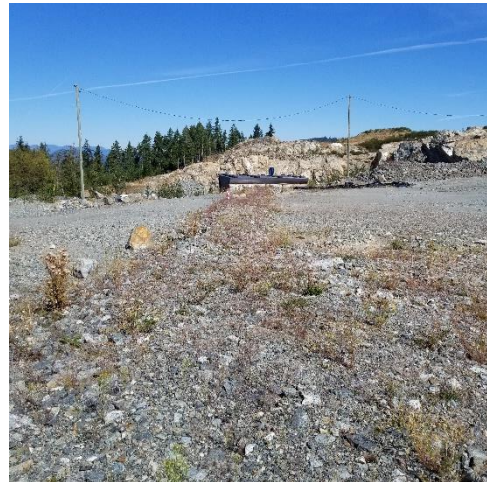
Leak and leachate detection works
