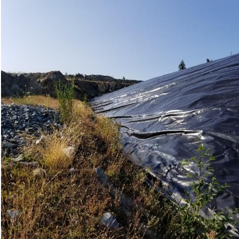
PEA – liner near NE corner
