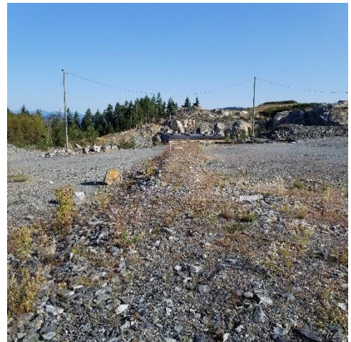
Leak and leachate detection works
