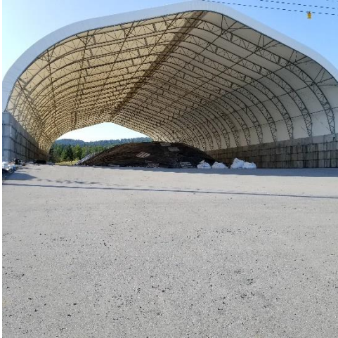
SMA - looking south
