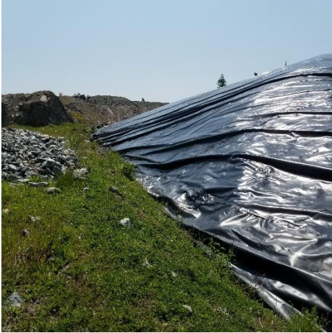
PEA – liner near NE corner
