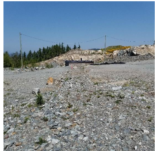
Leak and leachate detection works
