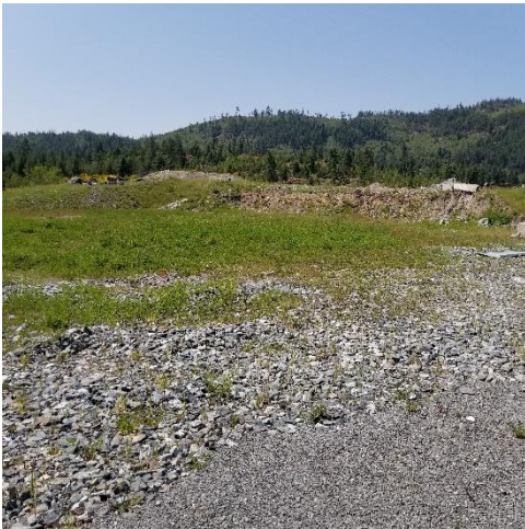
Contact water containment Pond
