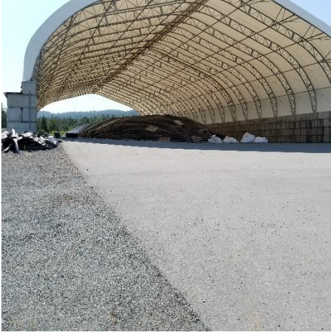
SMA - looking south
