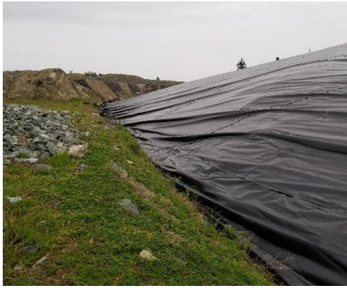
PEA – liner near NE corner
