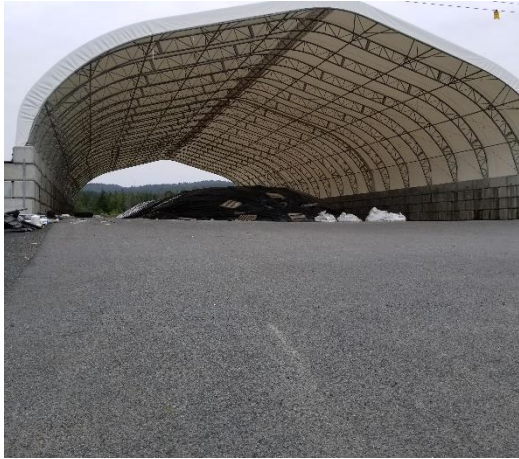
SMA - looking south
