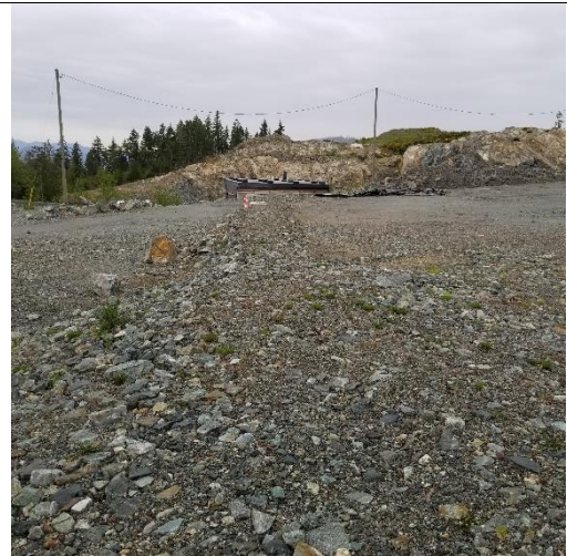
Leak and leachate detection works
