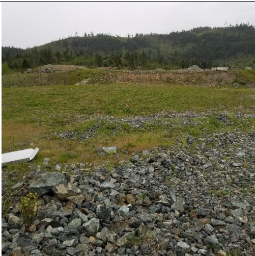
Contact water containment Pond
