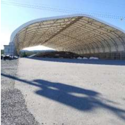
SMA - looking south
