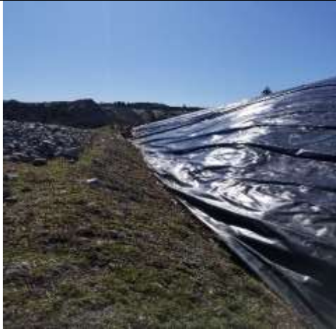
PEA – liner near NE corner
