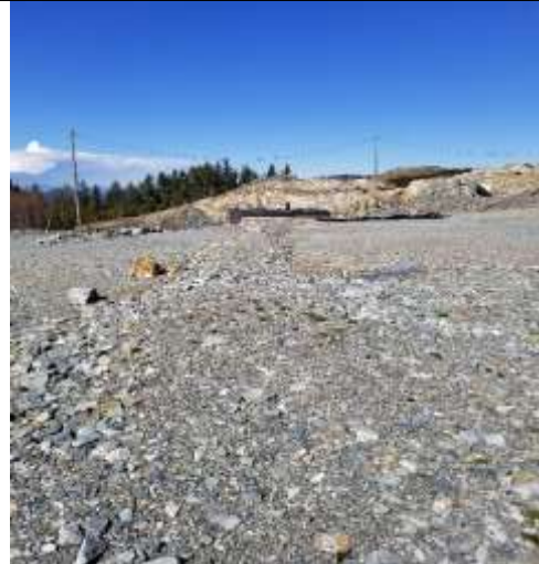
Leak and leachate detection works
