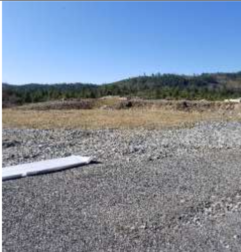
Contact water containment Pond
