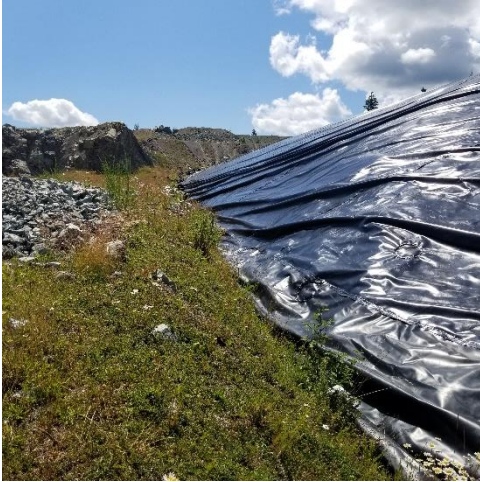
PEA – liner near NE corner
