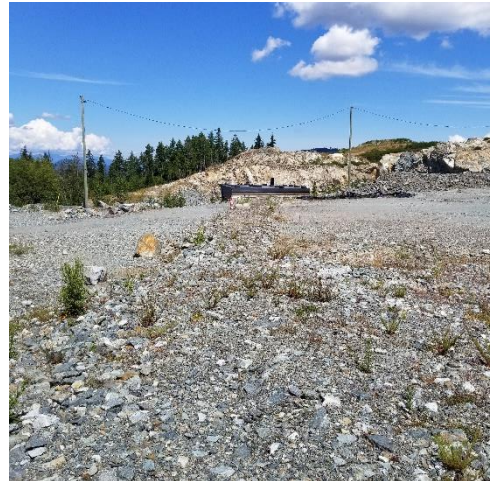
Leak and leachate detection works
