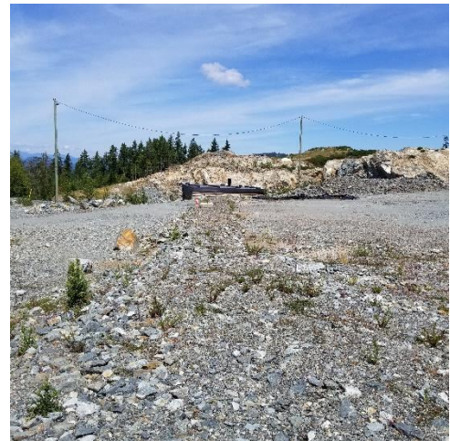
Leak and leachate detection works
