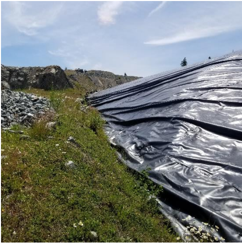
PEA – liner near NE corner
