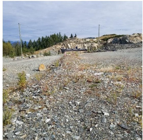
Leak and leachate detection works
