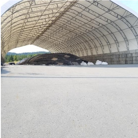
SMA - looking south
