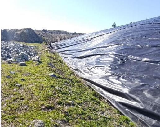
PEA – liner near NE corner
