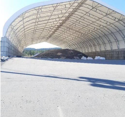
SMA - looking south
