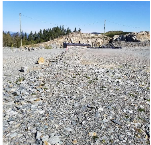
Leak and leachate detection works
