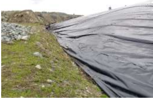
PEA – liner near NE corner
