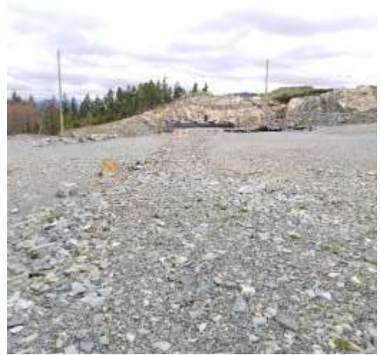
Leak and leachate detection works
