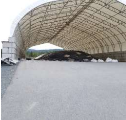
SMA - looking south
