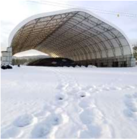
SMA - looking south
