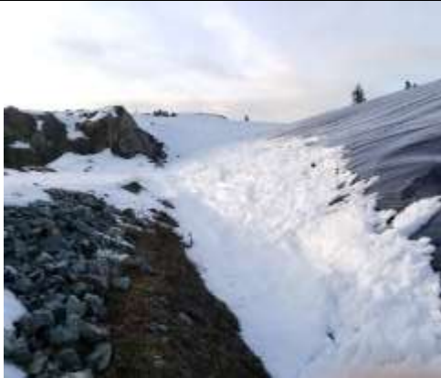
PEA – liner near NE corner
