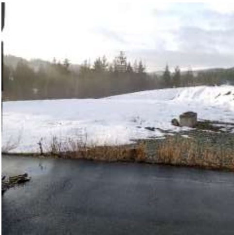
Contact water containment Pond
