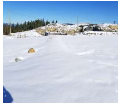
Leak and leachate detection works
