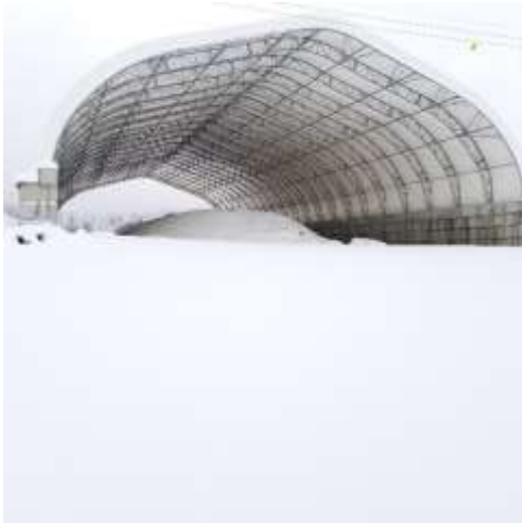
SMA - looking south
