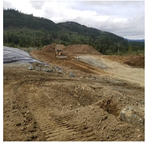
Stockpile Location – Looking West
