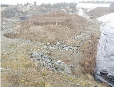
Site – Looking East
