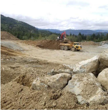
Stockpile Location – Looking Northwest
