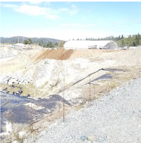
Stockpile Location – Looking Northeast
