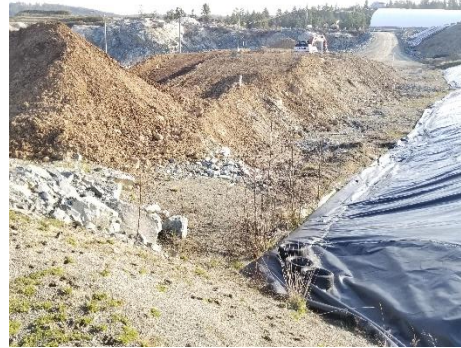
Stockpile Location – Looking East
