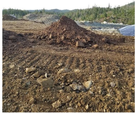
Soil Stockpiling – Looking South
