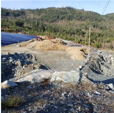
Site – Looking West
