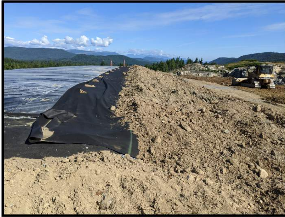
Picture # 5: Construction of cap along eastern PEA face has reached peak of PEA liner.
