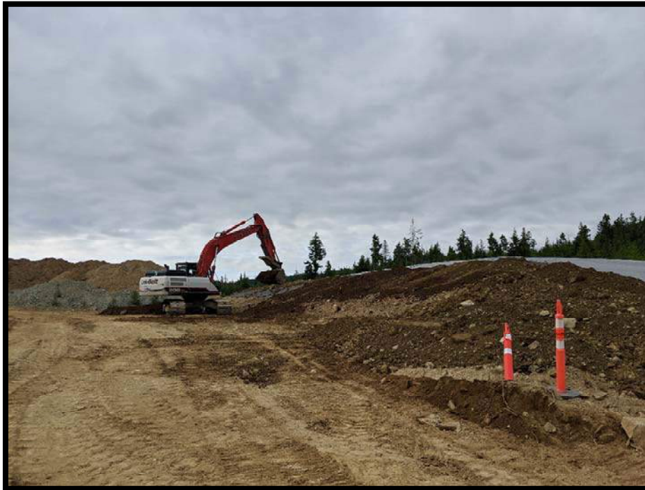
Picture # 3: Looking south along the east side of the PEA towards an excavator placing backfill material onto previously placed geofabric and drain rock..
