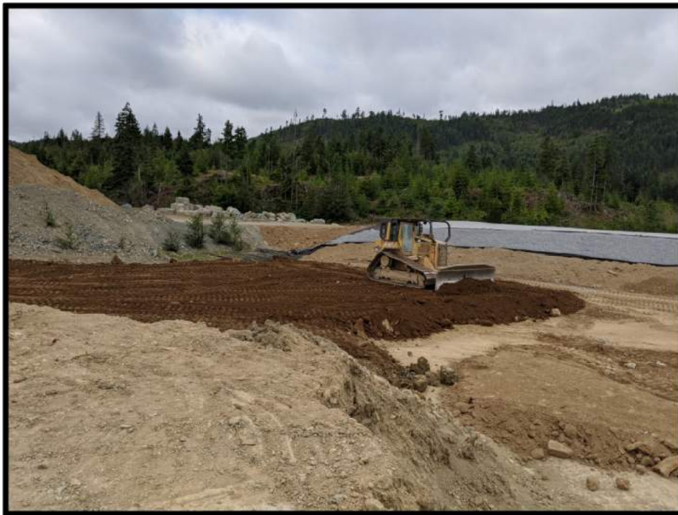
Picture # 4: D6 dozer spreading and compacting general fill east of PEA.
