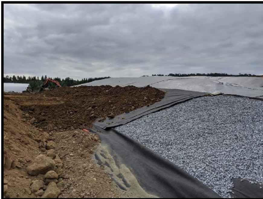
Picture # 3: Looking south along the east side of the PEA towards an excavator placing backfill material onto previously placed geofabric and drain rock..
