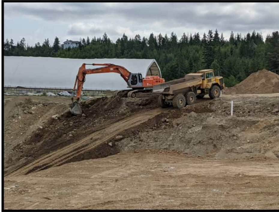
Picture # 5: Contractor moving stockpiled soils to PEA slope with rock truck.
