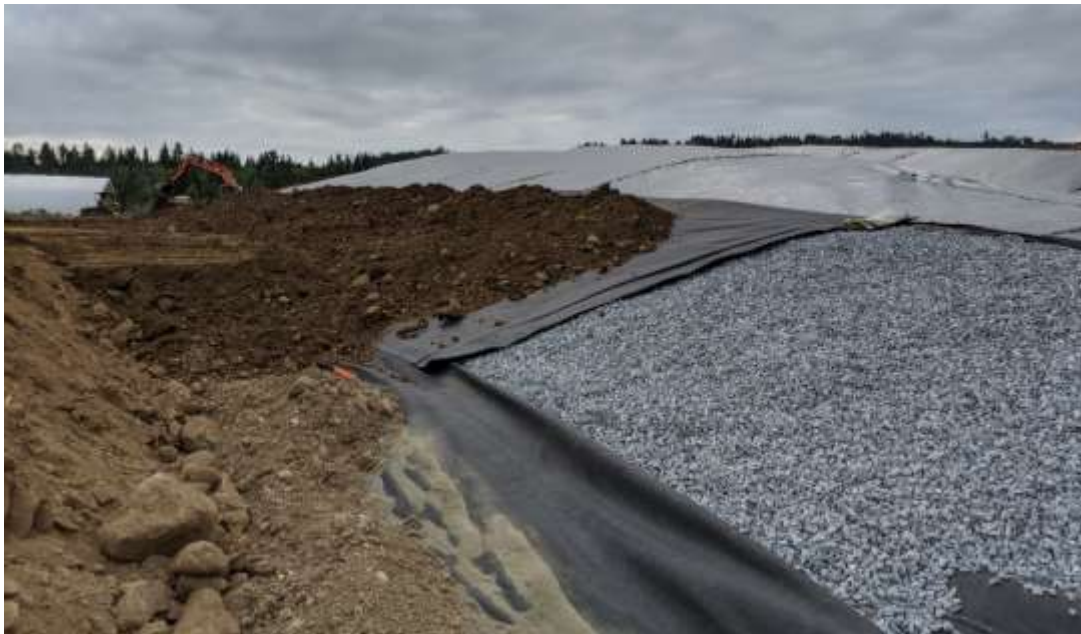
Picture #2: Placement of Closure Layers on the PEA
