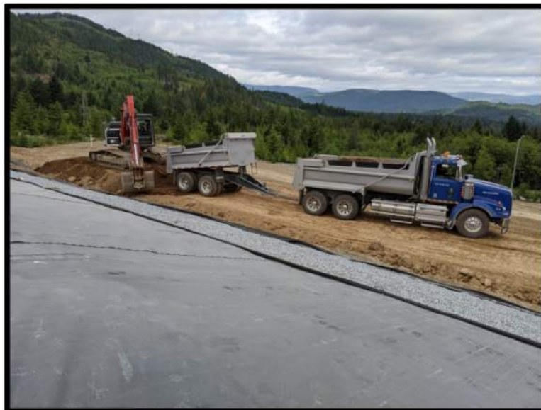
Picture # 6: Import soils from 2251 Bear Mountain deposited at northern slope of PEA.
