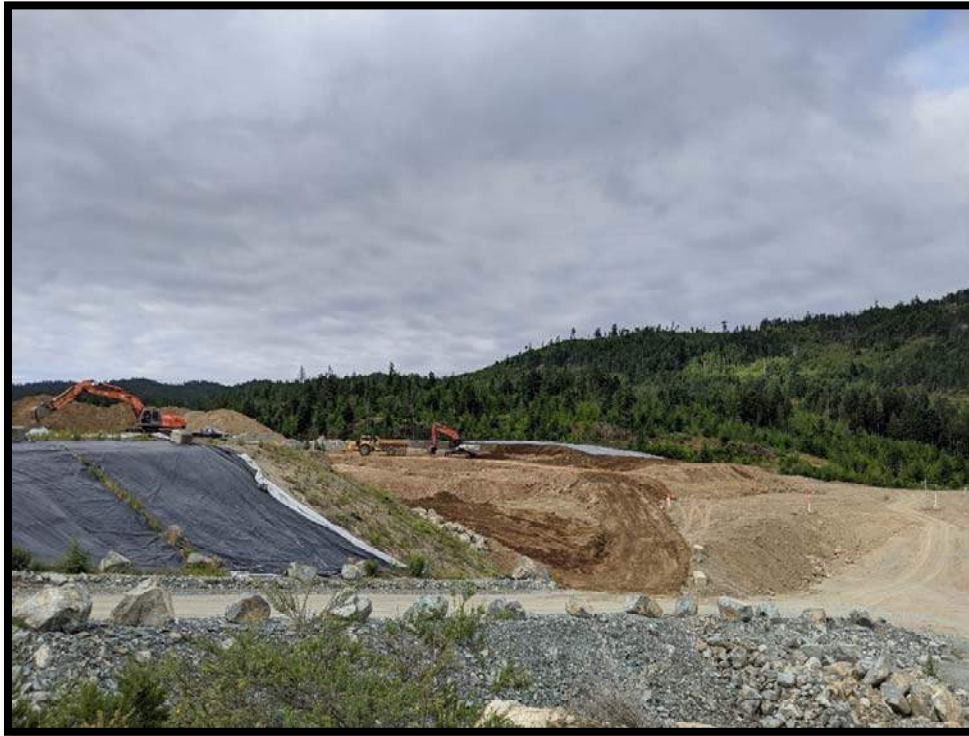
Picture # 1: Overview of construction progress, looking west.
