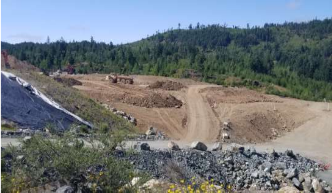
Picture #1: Looking Southwest at the PEA
