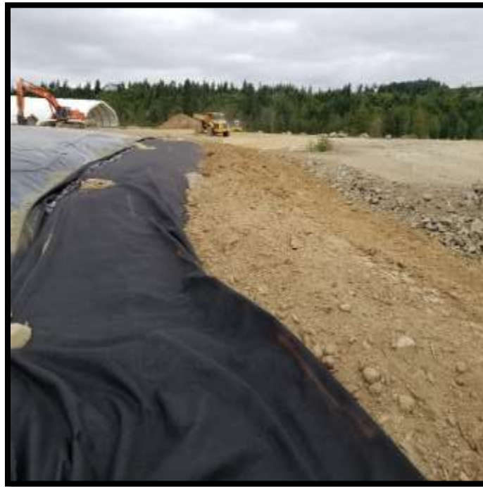
Picture # 5: Truck Ramp to PEA South Crest – Looking East
