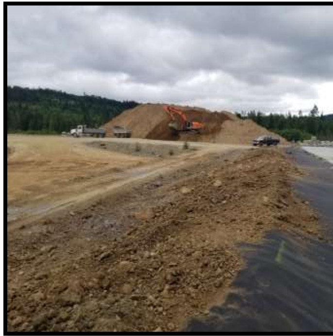
Picture # 5: Stockpile Location – South Stockpile
