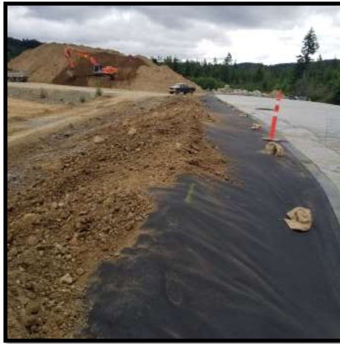
Picture # 3: Soil Placement to Crest on the East Face – Looking South
