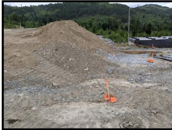
Picture # 1: Contractor has laid out toe of slope for PEA cover..
