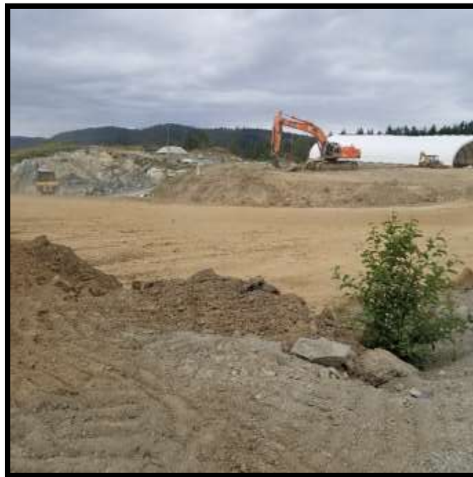
Picture # 4: Soil Movement From the East Stockpile to the PEA Slopes
