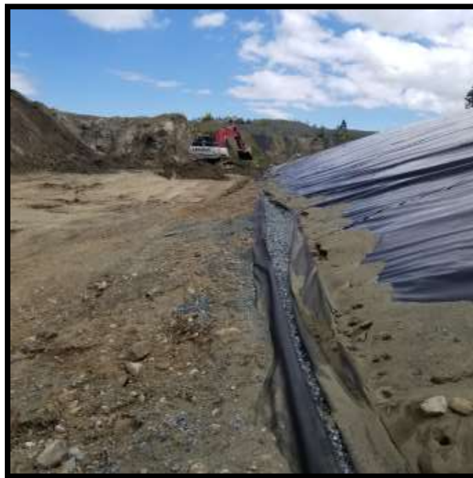
Picture # 6: PEA East drainage trench – Method – Soil Placement over drainage material layers.
