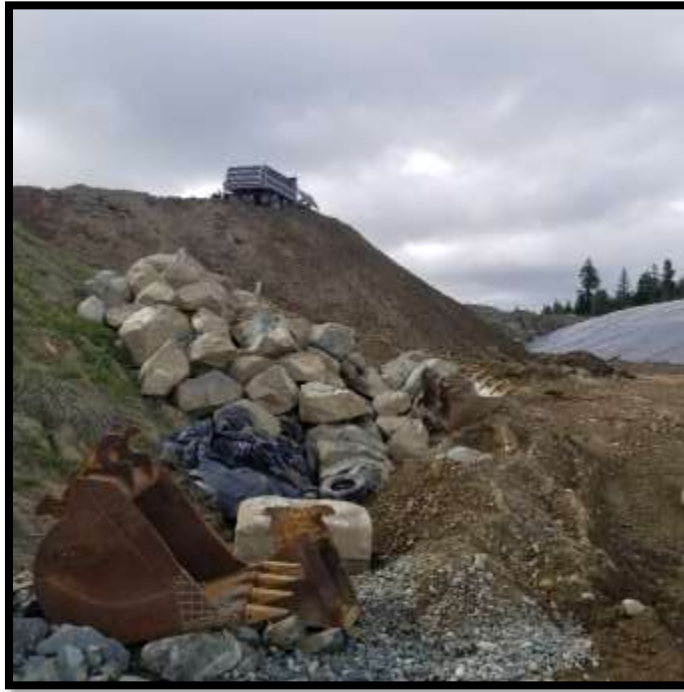
Picture # 1: Stockpile Location – East Stockpile.
