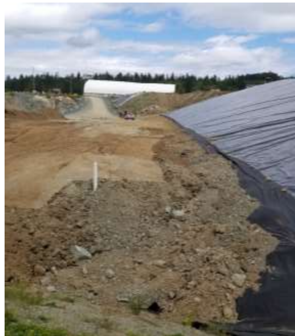
Photo 3: Looking east at common fill stabilizing wedge at north side of PEA
