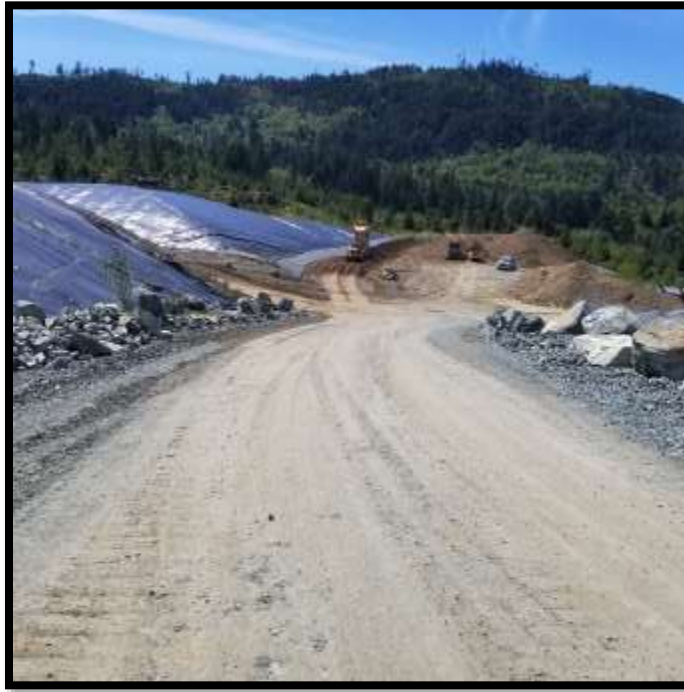
Picture # 1: Imported material is used to build a truck ramp outside of the PEA North toe.
