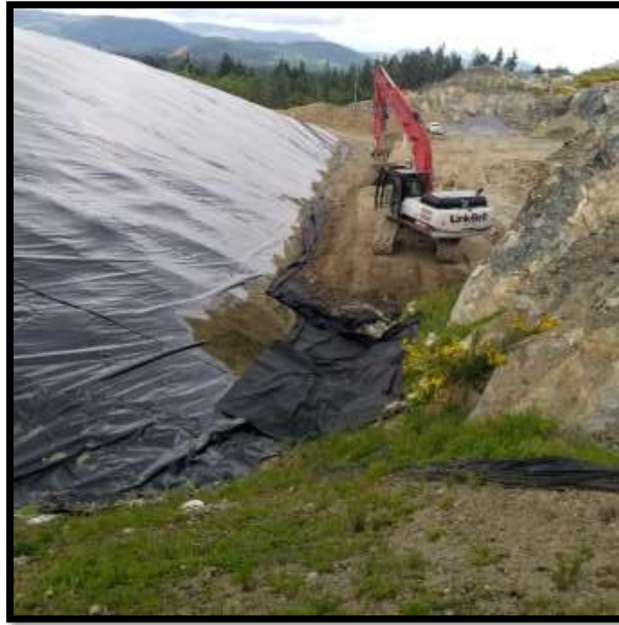
Picture # 3: PEA drainage trench coverage – Looking North
