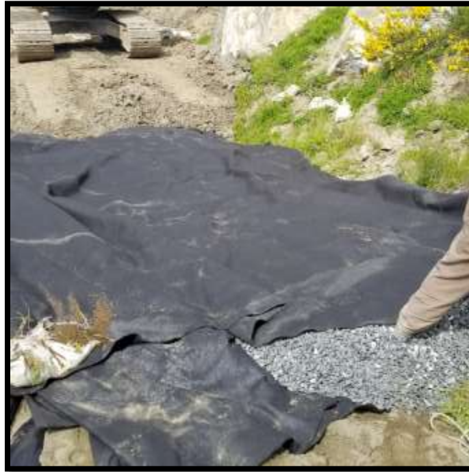
Picture # 5: PEA East drainage trench – Method – Gravel placement over geotextile, rock, geotextile, sand layers.
