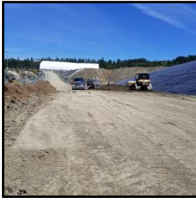
Picture # 1: Stockpile Location – PEA Northeast Toe.
