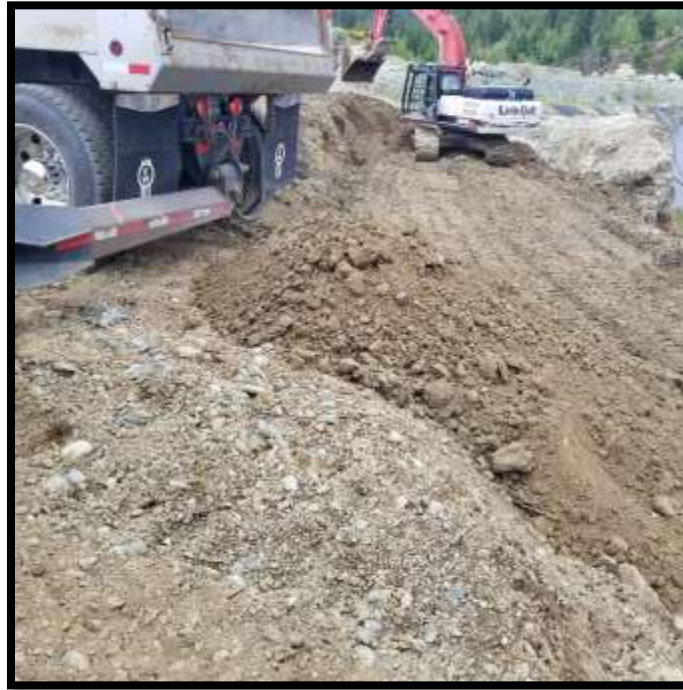
Picture # 1: Imported material stockpiled at the East stockpile location – New source material is from Admirals Road/McKenzie Interchange Phase 2 construction
