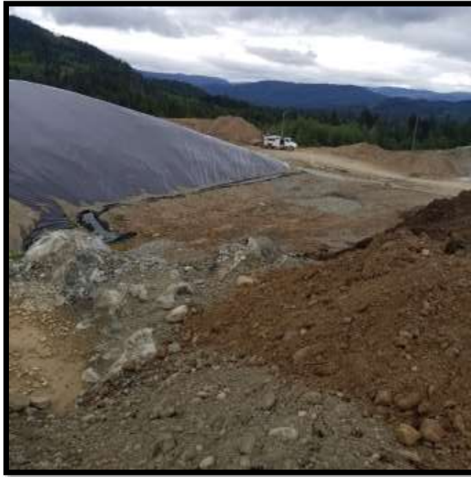
Picture # 3: PEA East trench coverage – Looking Northeast.
