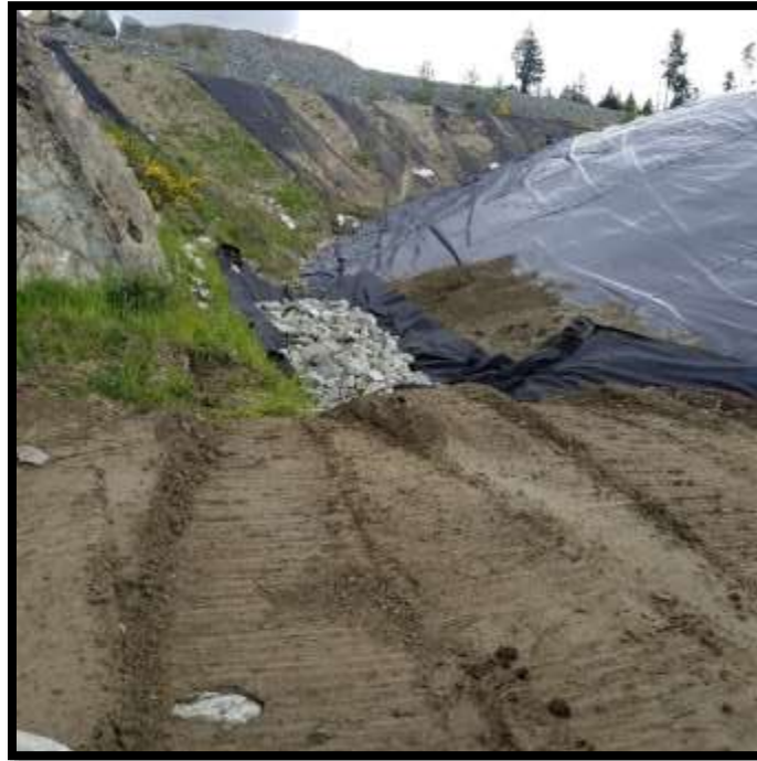
Picture # 4: PEA drainage trench coverage – Method – Rock Placement over sand and geotextile.
