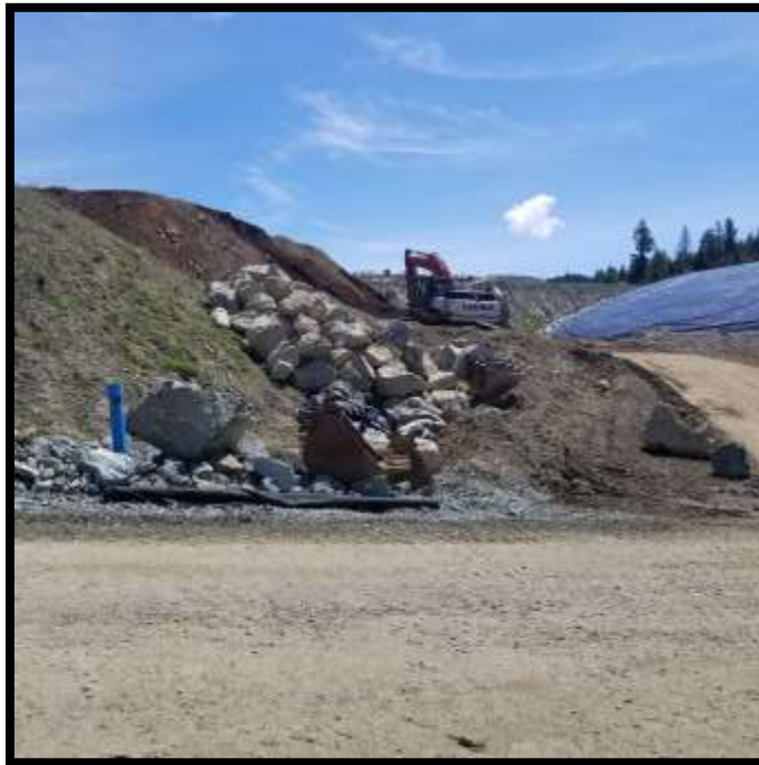
Picture # 2: Soil from the East stockpile was used for the truck ramp.
