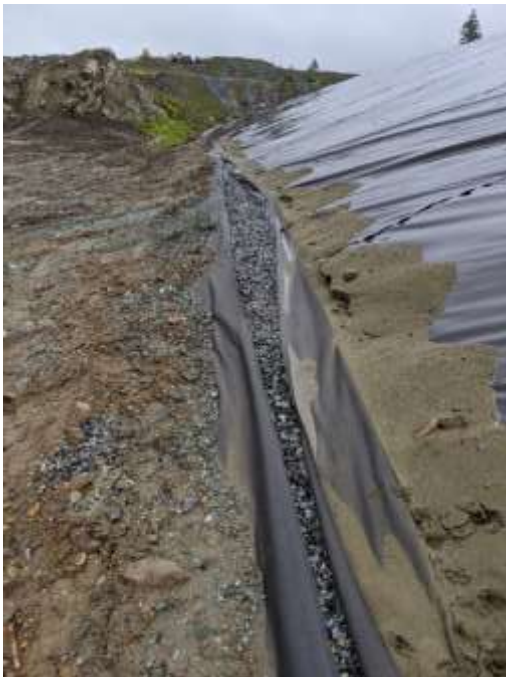
Photo 2: Cover Layers: Sand, 12 oz. geotextile, drainage gravel, 8 oz. geotextile, and common fill on north slope of PEA
