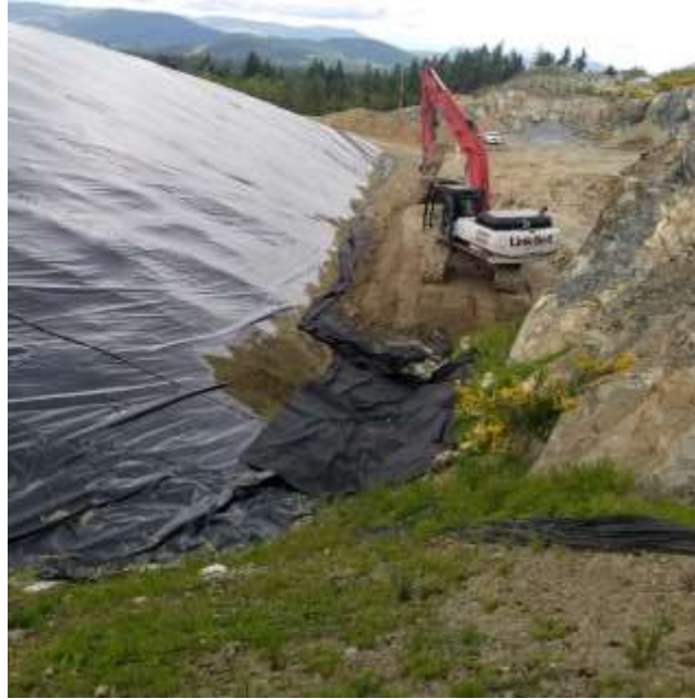
Photo 1: Alterra covering PEA toe drainage soakaway trench on east side of PEA
