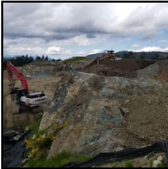
Picture # 2: A pad is built surrounding SB4.
