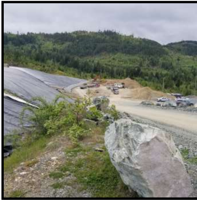
Picture # 4: Soil dump location adjacent to PEA North toe.
