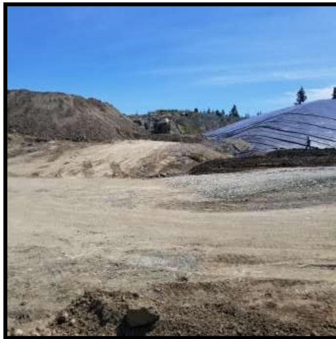
Picture # 2: Stockpile Location – PEA East Toe.
