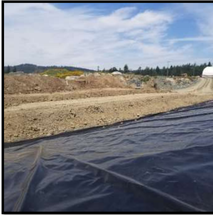
Picture # 3: Stockpile Location – PEA North Toe – Looking Northeast.
