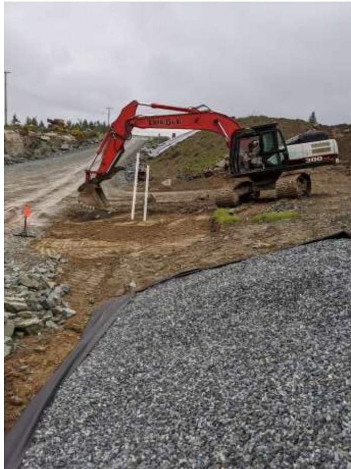
Photo 4: Cleanout Extensions on east side of PEA
