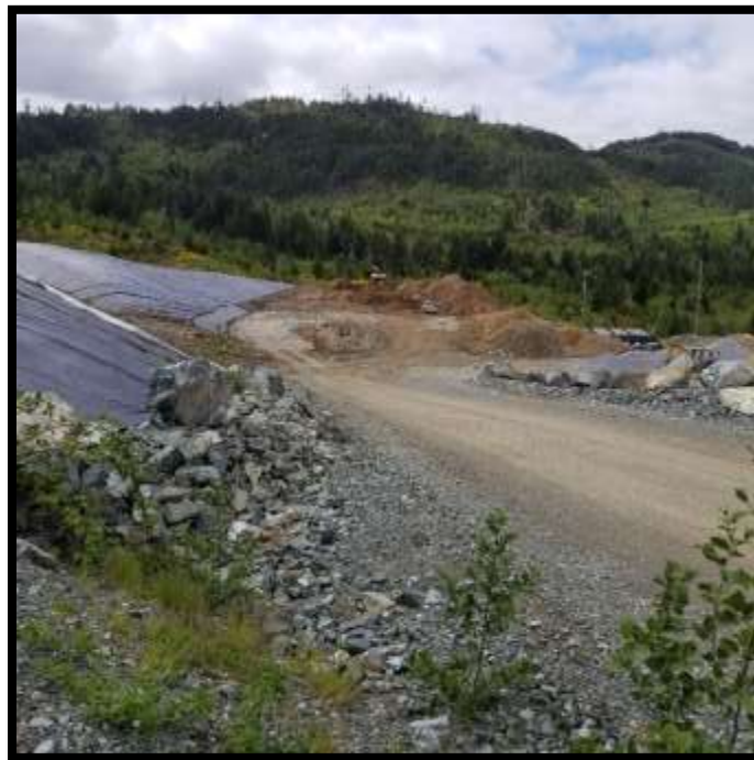
Picture # 2: PEA North toe trench coverage.
