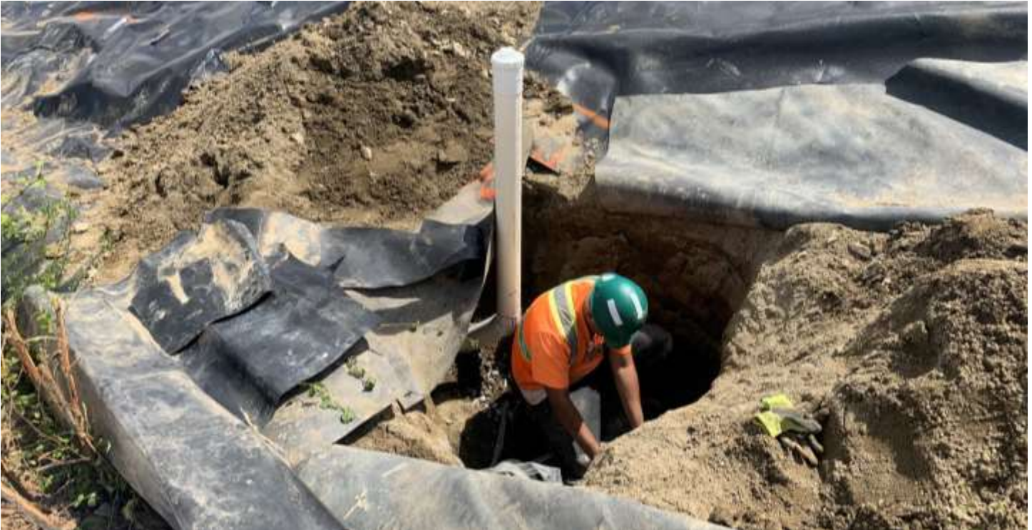
Picture # 5: Allterra located the leachate collection pipe on the west side and installed cleanout pipe extension .
