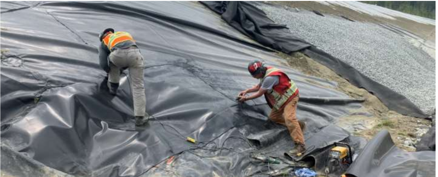
Picture # 1: Western Tank & Lining (WTL) was on-site to install patches and boots on the areas where the PEA geomembrane was cut to expose the leachate collection pipes.
