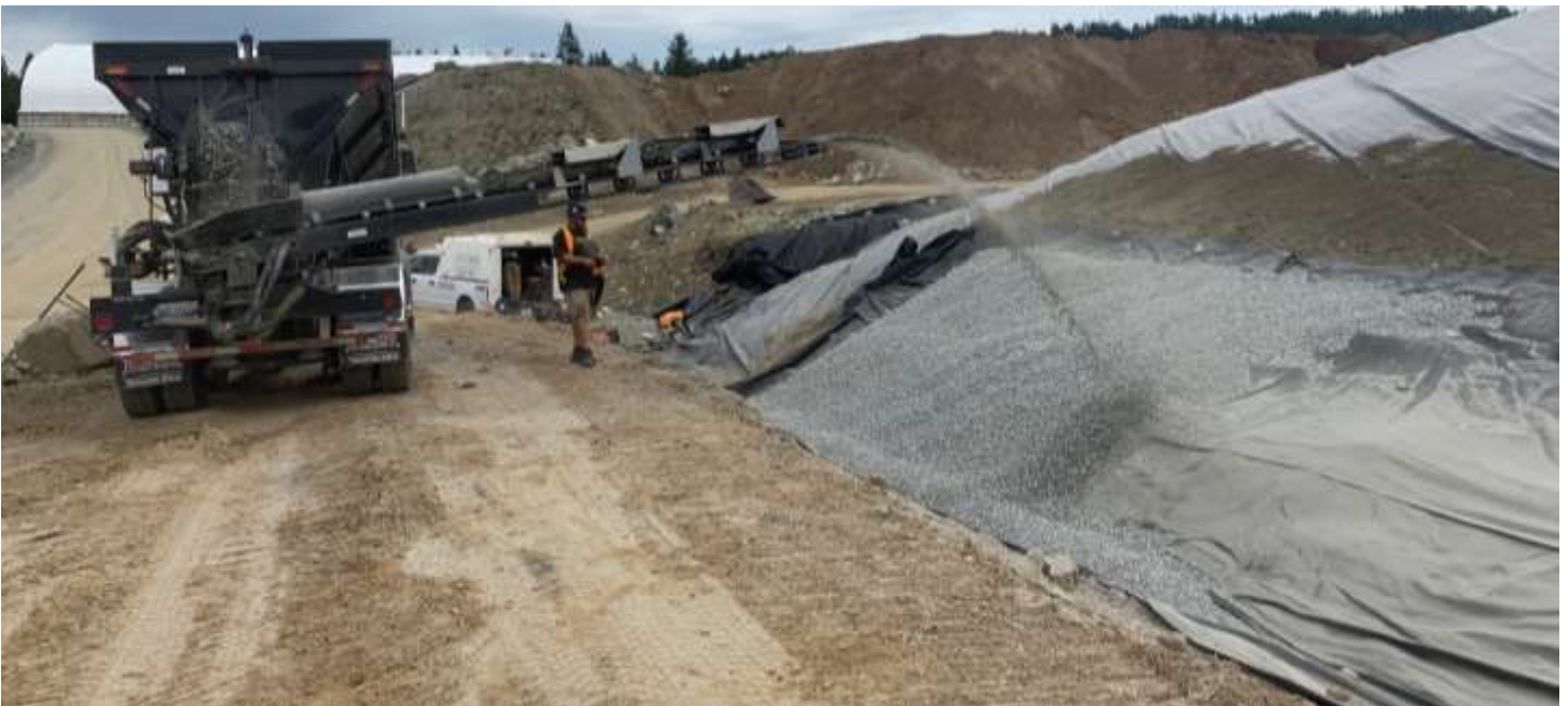
Picture # 8: Allterra used a stone slinger to place 200 mm thick layer of 5 to 25 mm clear crush drainage gravel on the PEA north side slopes above the 12 oz. geotextile.
