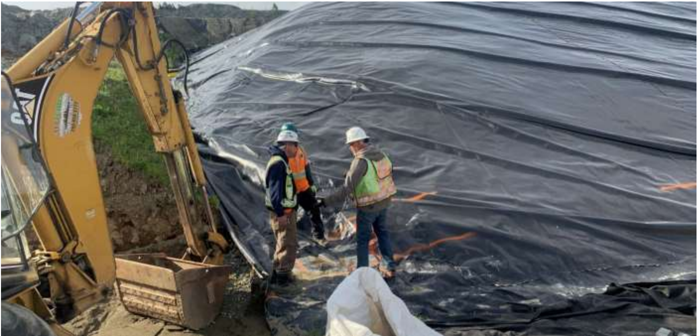
Picture # 1: Looking at east side of Permanent Encapsulation Area (PEA). Allterra's goal for the day was to locate and expose the existing leachate collection and sub liner leak detection pipes to install a total of four (4) cleanouts. Refer to attached Figure 4-6 for cross section showing detail for leachate collection and leak detection piping.
