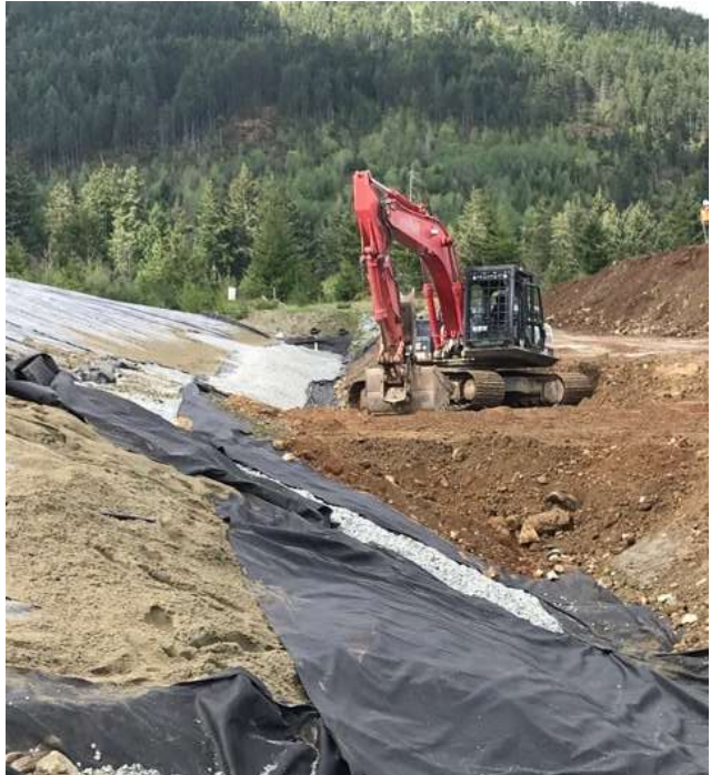
Picture #7 : Allterra placed and compacted common fill against PEA slope to secure sand blanket and cover layers. Geotextile intentionally peeled back to show underlying gravel layer
