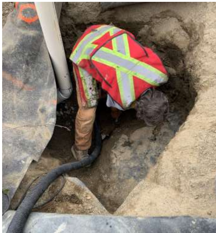
Picture # 4: WTL tech used a vacuum to remove small amount of water pooled below the invert of the leachate collector pipe at the west leachate collector cleanout so that WTL could repair liner hole on the bottom liner.
