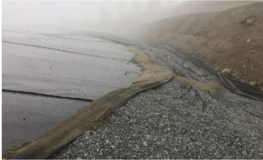
Picture #5: On May 12, 2020 there was a small rain induced failure of the sand blanket on the north slope of the PEA, which Allterra repaired.
