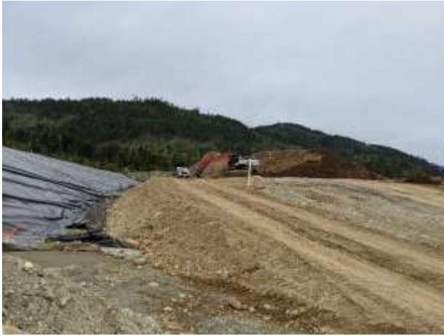
Picture #2: Looking west at common fill at toe of PEA
