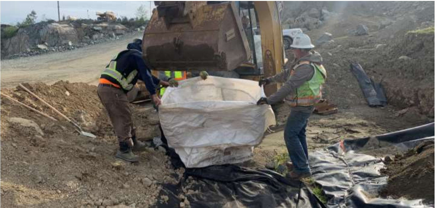
Picture # 3: Allterra excavated out the material located under the PEA cover geomembrane in the exposed areas. All excavated soil was either backfilled under the PEA geomembrane or placed into mega bags and stored in the Soil Management Area (SMA).
