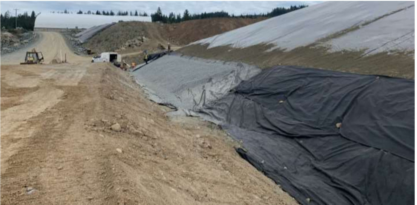
Picture # 9: North side slope of PEA with 5-25 mm drainage gravel layer, geotextile, and sand layer installed.
