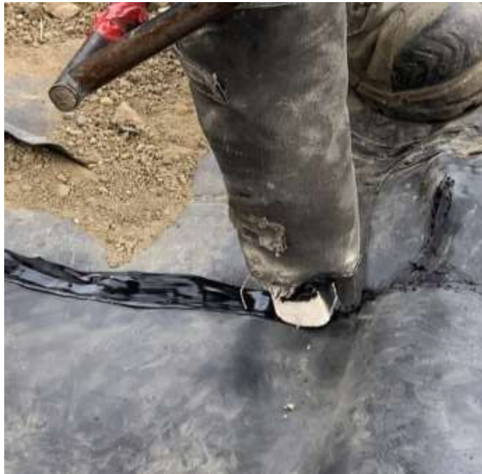
Picture # 3: Close up of WTL extrusion welding patch on PEA geomembrane.
