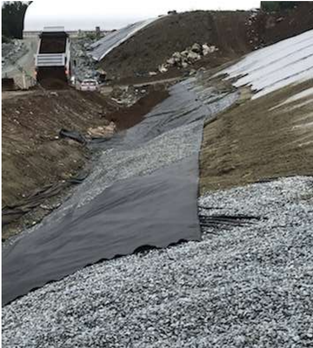
Picture #6: Allterra repaired sand blanket and deployed 12 oz. geotextile and drainage gravel
