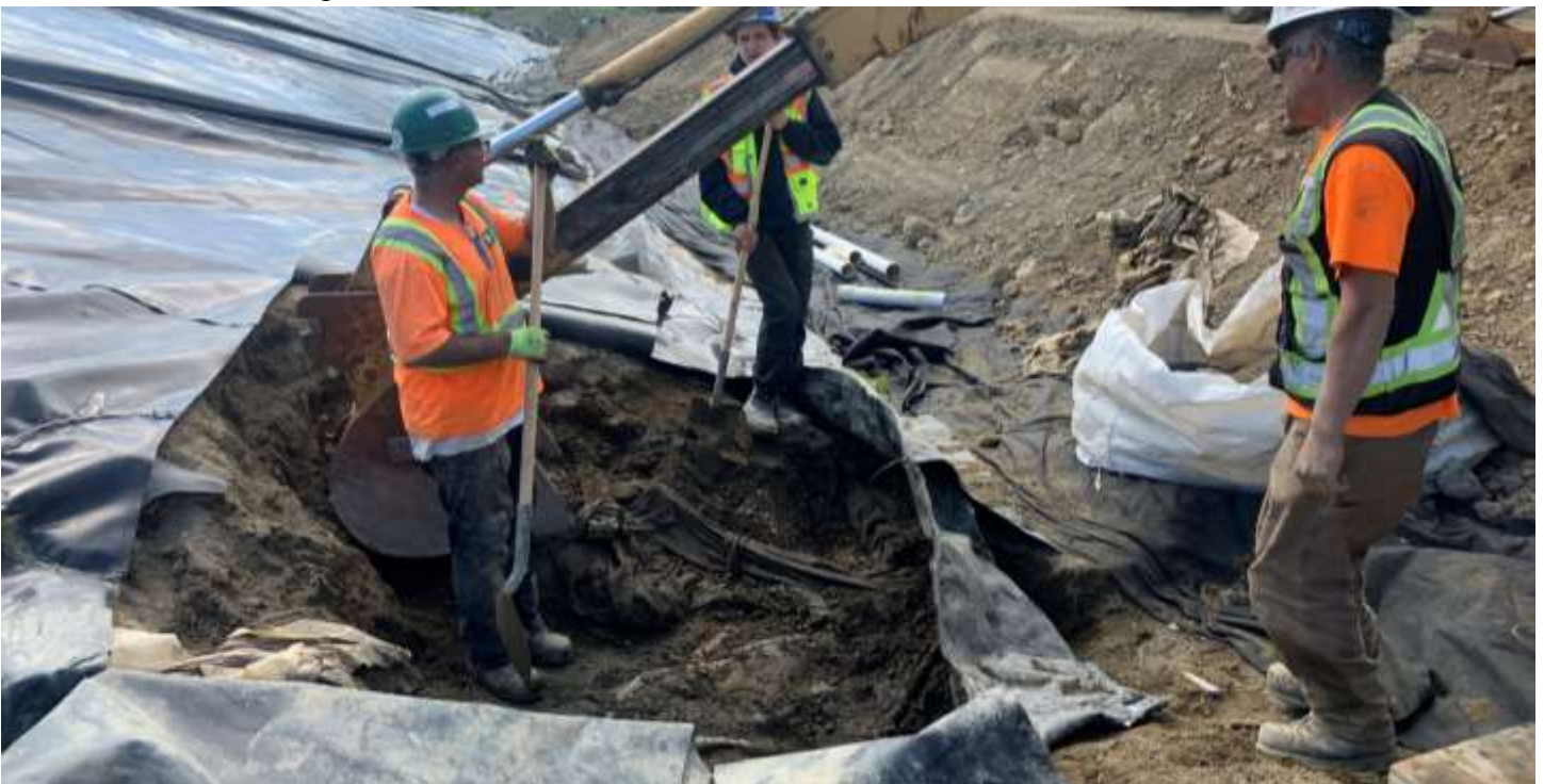
Picture # 4: Allterra located the leachate collection pipe on the east side. Allterra also hand excavated material and exposed the leak detection pipe located under the basal liner.
