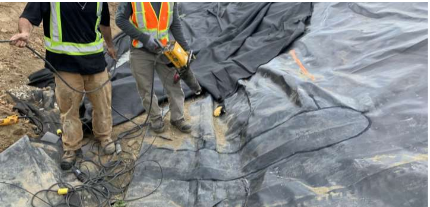
Picture # 2: WTL installing patch on PEA geomembrane with extrusion welding machine.
