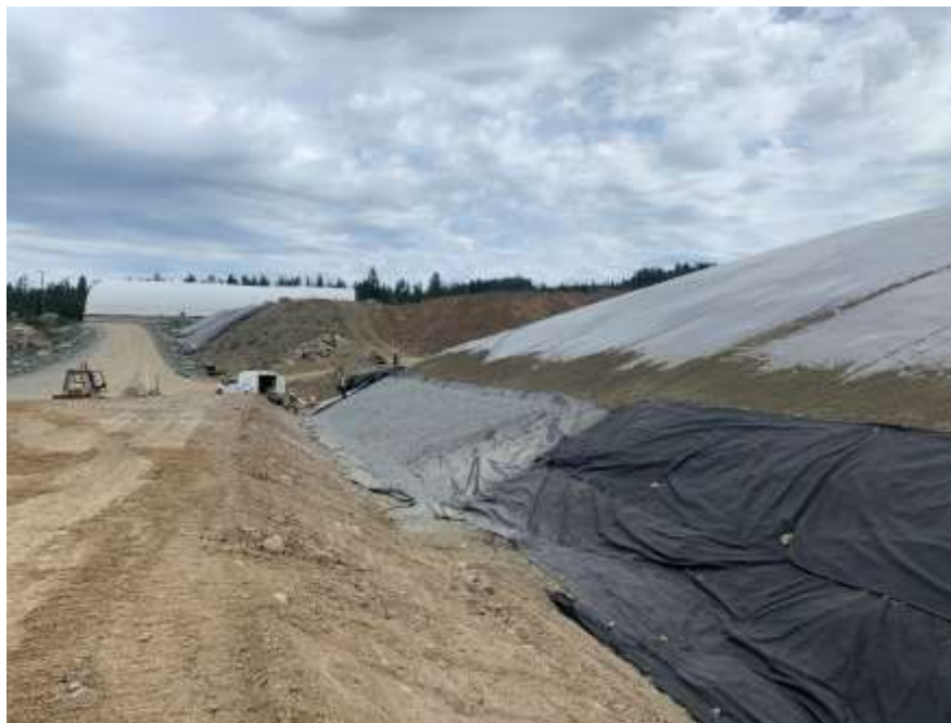
Picture #4: Looking east at north slope of PEA. Sand blanket, 12 oz. geotextile, and drainage gravel installed on lower north slope.
