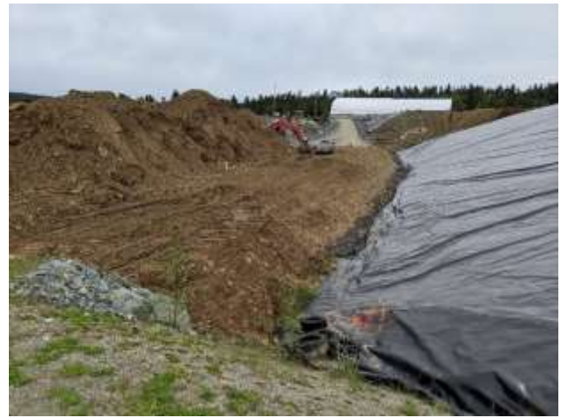
Picture #3: Looking east at common fill at toe of PEA
