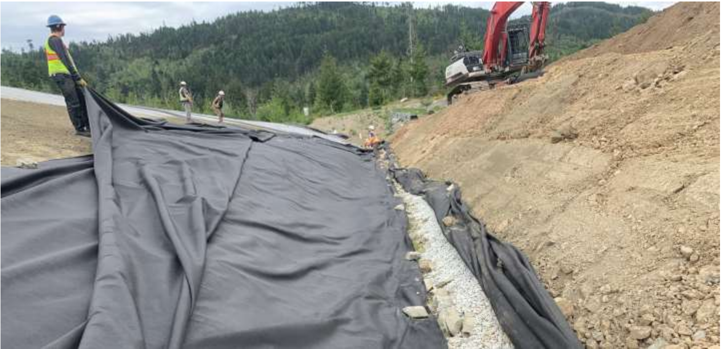
Picture # 7: Allterra workers stretching lower geotextile on east edge of PEAso a stone slinger can place gravel layer (min. 200 mm thick) on PEA north side slopes over the sand layer.
