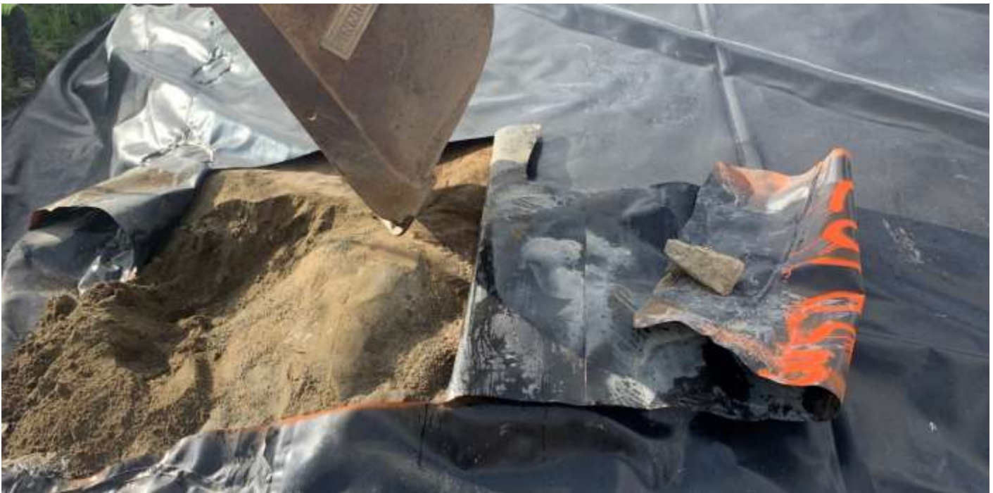
Picture # 2: Allterra cutting hole in PEA geomembrane on east side to expose existing leachate collector pipe to install cleanouts.
