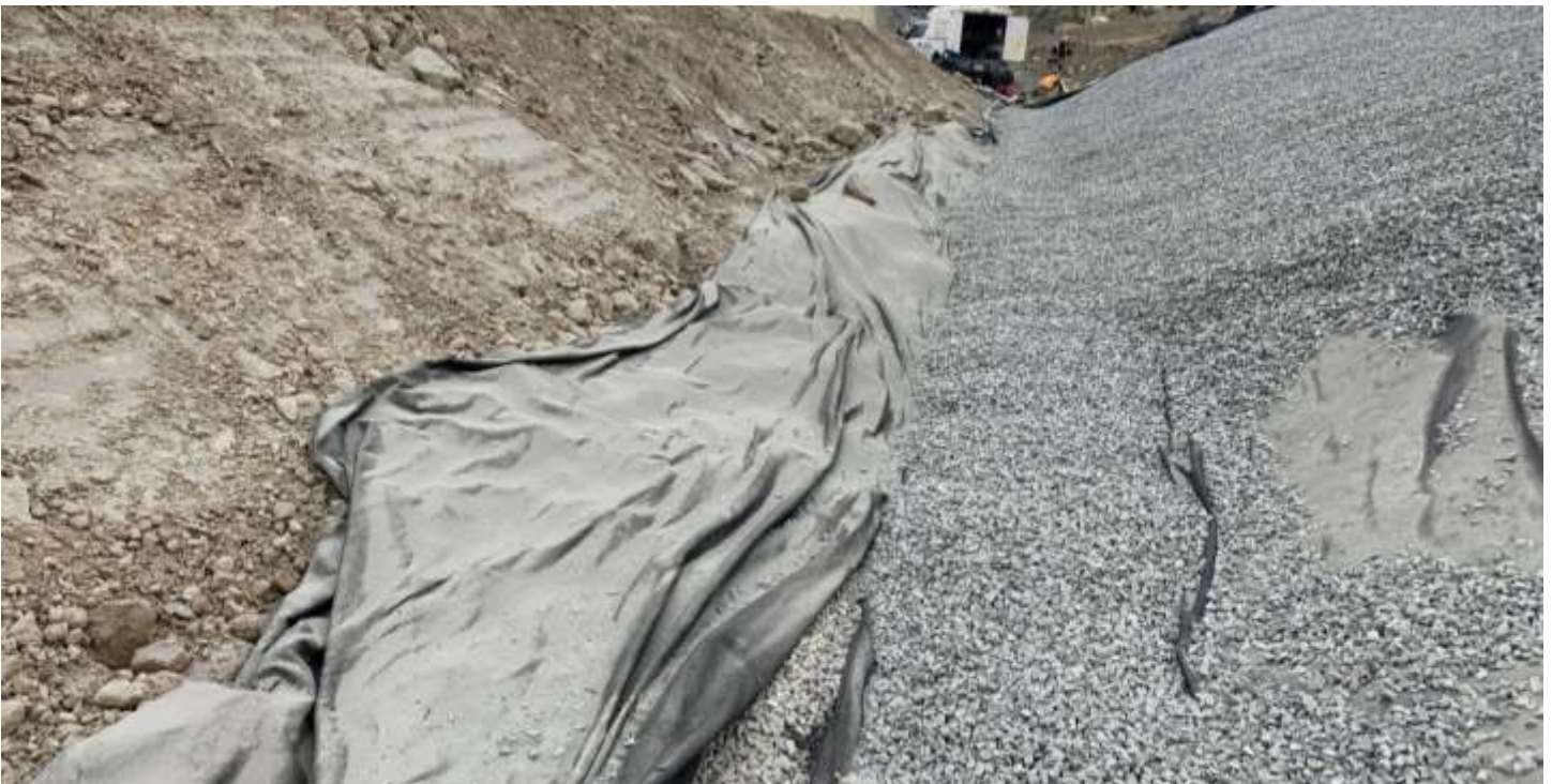
Picture # 10: Allterra ensured direct hydraulic contact between drainage gravel on side slopes and soak away trench at north toe of the PEA.
