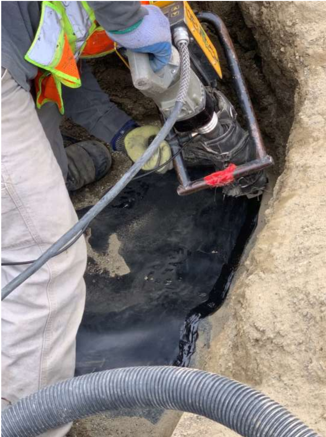
Picture # 5: WTL extrusion welding patch on bottom liner at west cleanout area.
