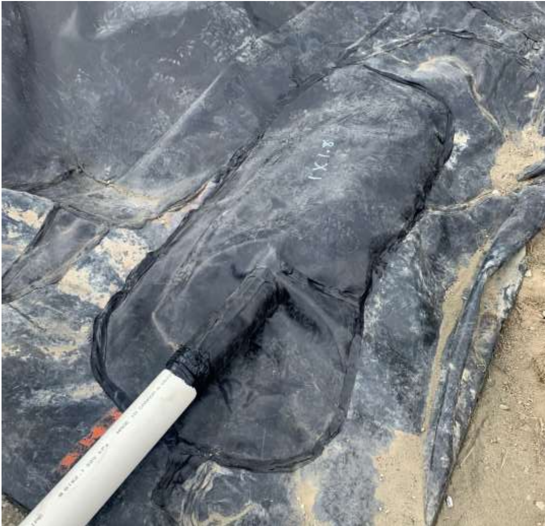
Picture # 6: WTL completed pipe liner penetration boot on east side of PEA. All extrusion welds were inspected and tested.
