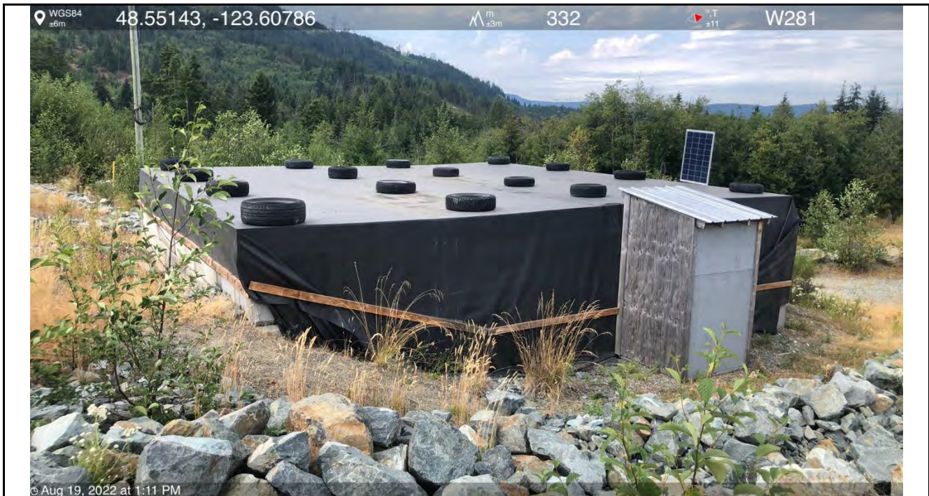
Photo 7: View of the south side of the storage tank facility looking west (August 19, 2022).
