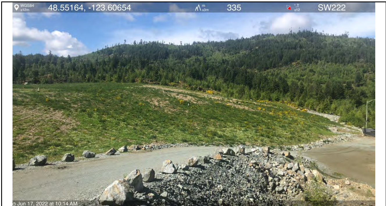
Photo 5: View of the PEA surface vegetation and scoured areas with little to no vegetation from the northeast corner looking southwest (June 17, 2022).
