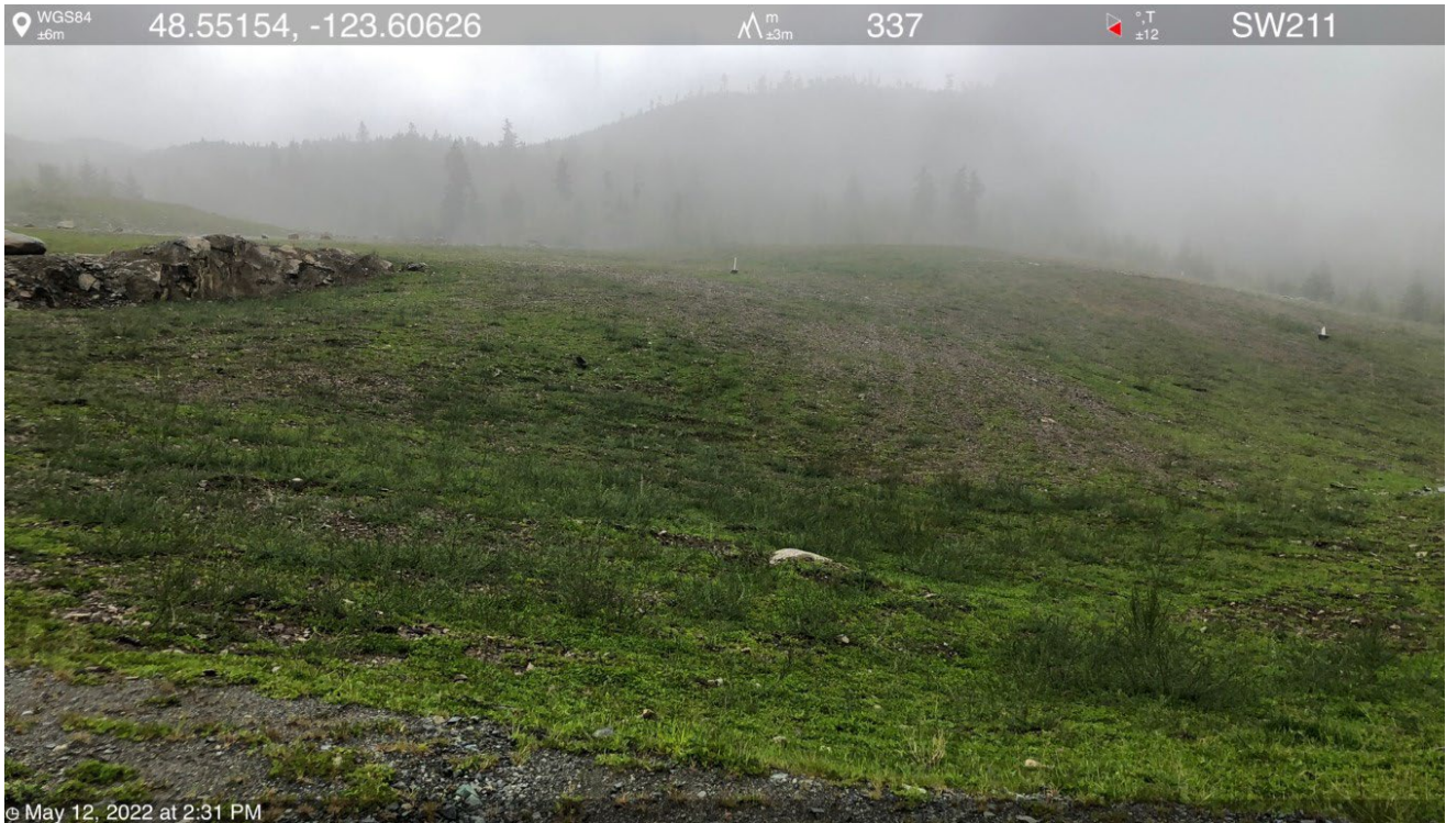
Photo 5: View of the PEA surface from the northeast corner looking southwest (May 2022).
