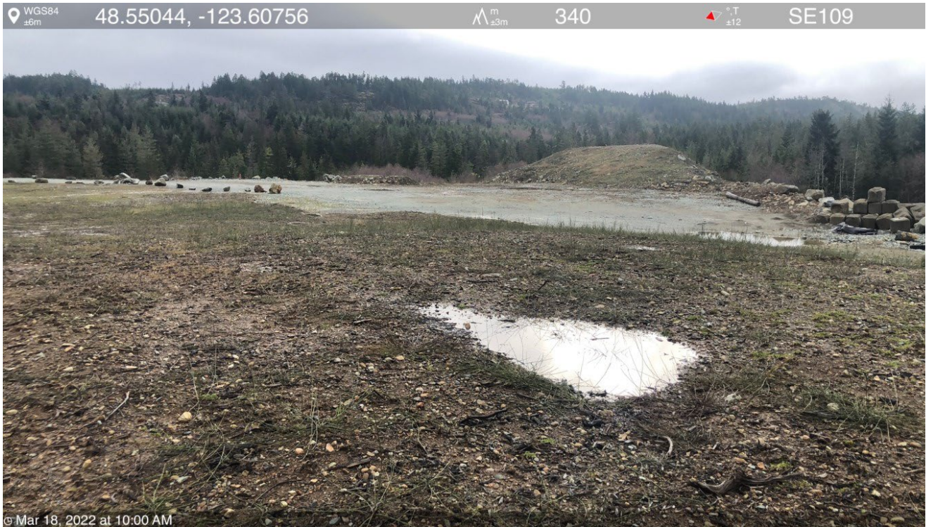
Photo 7: View of shallow standing water on the southern portion of the landfill cover looking southeast (March 2022).
