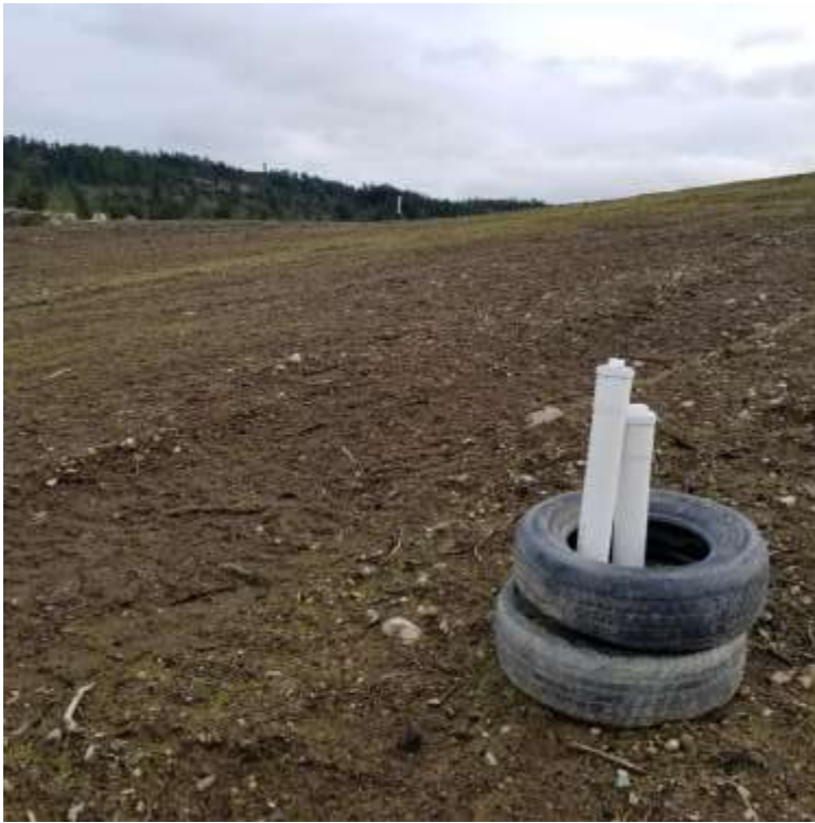
Picture #1: Groundwater monitoring well stand pipe
