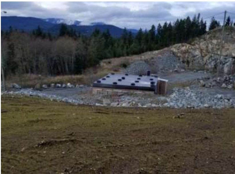
Picture #8: Leachate storage facility
