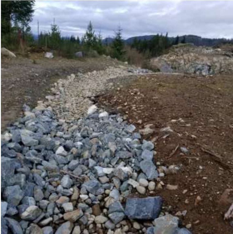
Picture #3: Surface water ditch on west crest
