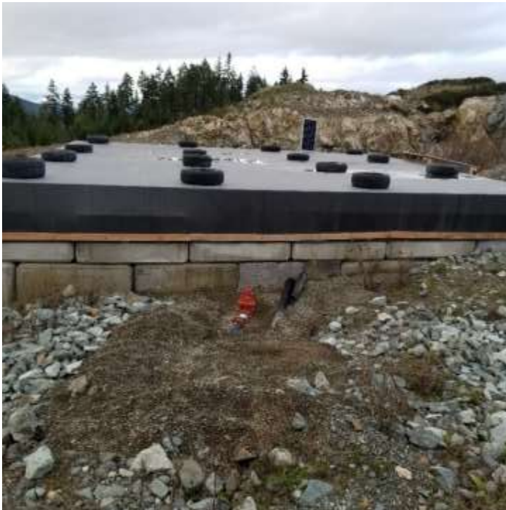
Picture #9: Leachate storage facility and valve
