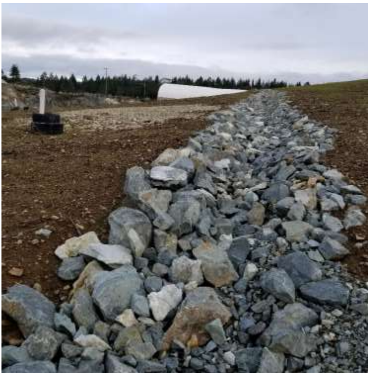
Picture #2: Surface water ditch on north crest
