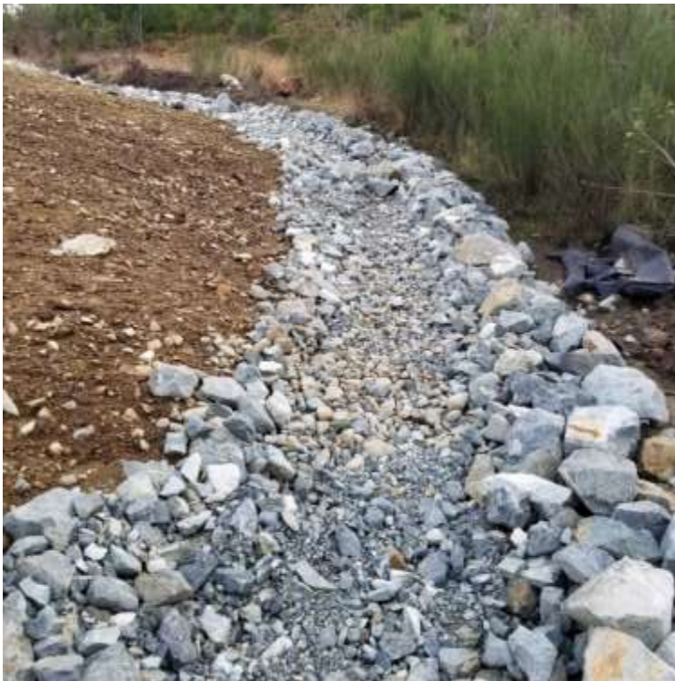
Picture #4: Surface water ditch on west crest
