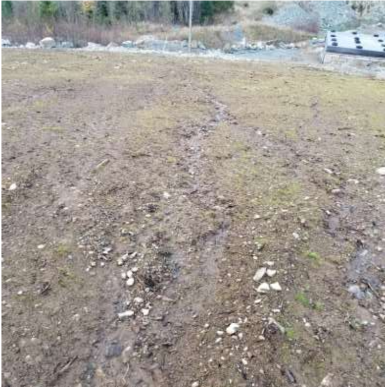
Picture #11: Mild erosion on north slope after large storm event
