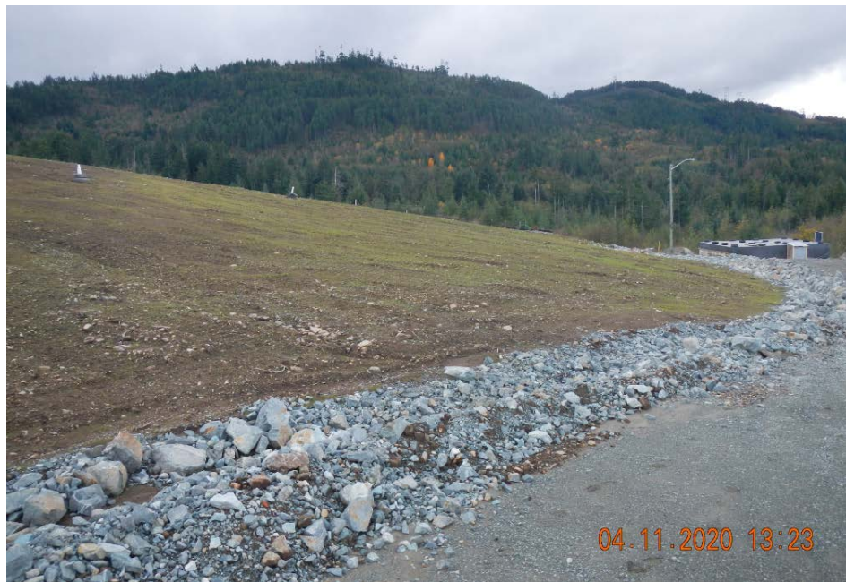
Photo 2 Revised south toe drainage trench
