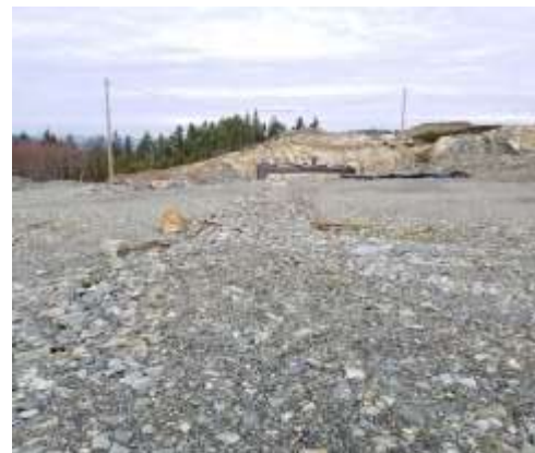
Leak and leachate detection works
