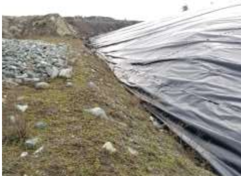
PEA – liner near NE corner
