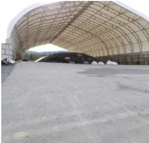
SMA - looking south
