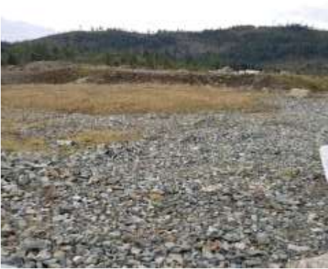
Contact water containment Pond
