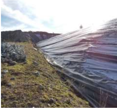
PEA – liner near NE corner
