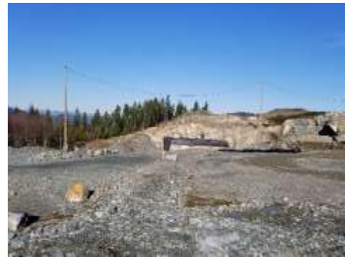
Leak and leachate detection works
