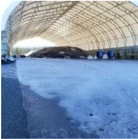
SMA - looking south
