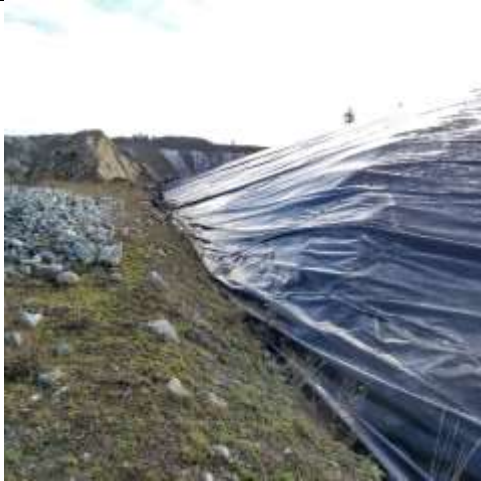
PEA – liner near NE corner
