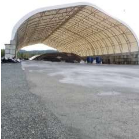
SMA - looking south
