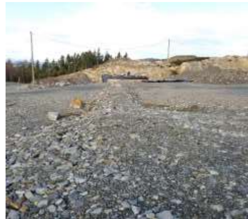
Leak and leachate detection works
