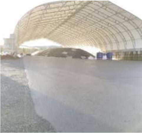
SMA - looking south
