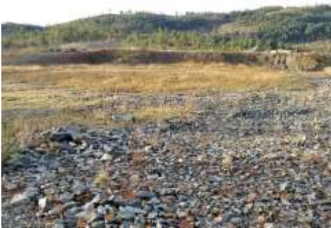
Contact water containment Pond
