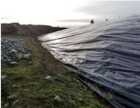
PEA – liner near NE corner
