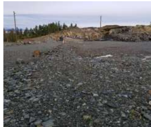
Leak and leachate detection works
