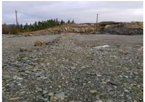
Leak and leachate detection works
