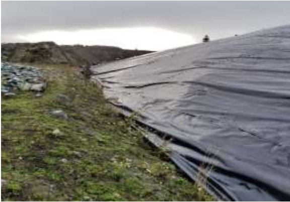
PEA – liner near NE corner
