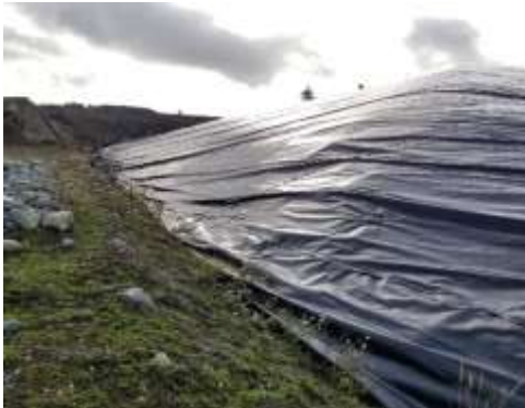
PEA – liner near NE corner
