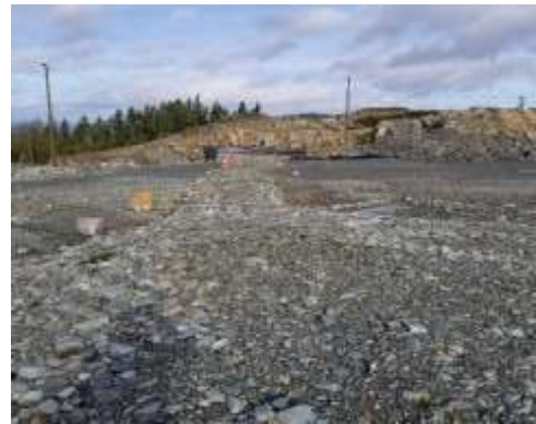
Leak and leachate detection works
