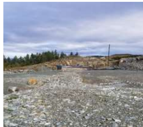
Leak and leachate detection works
