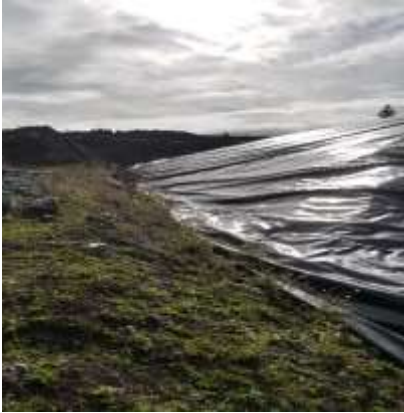
PEA – liner near NE corner
