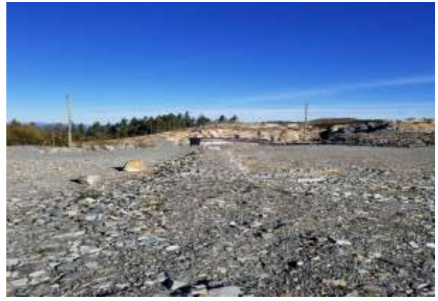
Leak and leachate detection works
