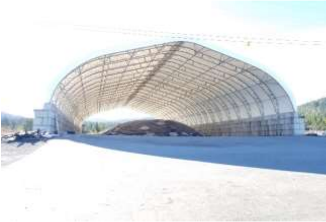
SMA - looking south
