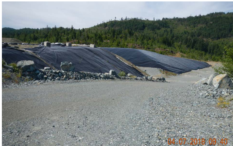
Photo 2 Looking west over clean soil (foreground, partially uncovered), and at northeast corner of sealed landfill
