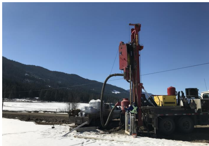
Figure 1: 2019 Hullcar Aquifer Monitoring Well Installation, Hullcar Aquifer
