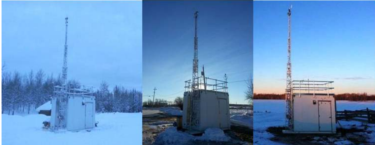
Figure 9 The three new ambient air quality stations installed in northeast BC. From left to right, Doig River station, Farmington station and Tomslake station. Each monitoring station was installed by the BC Ministry of Environment in December 2013 and January 2014 and contains instruments that measure concentrations of sulphur dioxide and total reduced sulfur. Both of these pollutants are associated with oil and gas development. Attached to each station is a ten metre high tower equipped with instruments measuring meteorological parameters including temperature, wind speed and direction.
