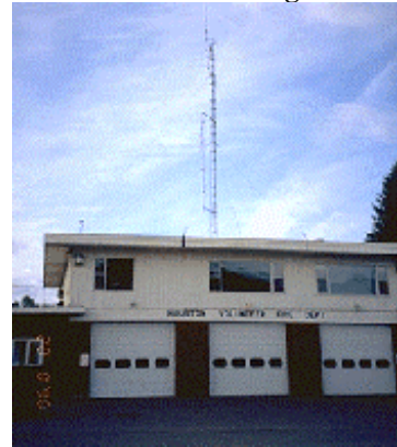
Figure 6. Firehall Monitoring Site
