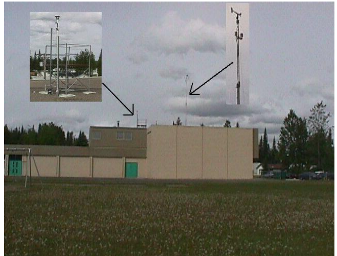
Glenview ambient and meteorological site looking towards the west
