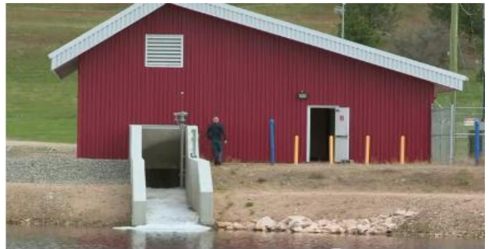
Photo: Lake Country Micro-Hydro Facility
