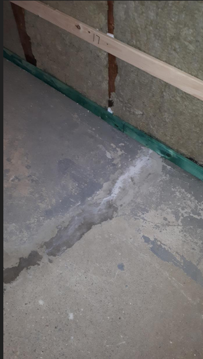
From Left: New wall with door frame and ceiling going in; Green waterproof sealant applied to wood; Cement cracks sealed prior to painting floor.
