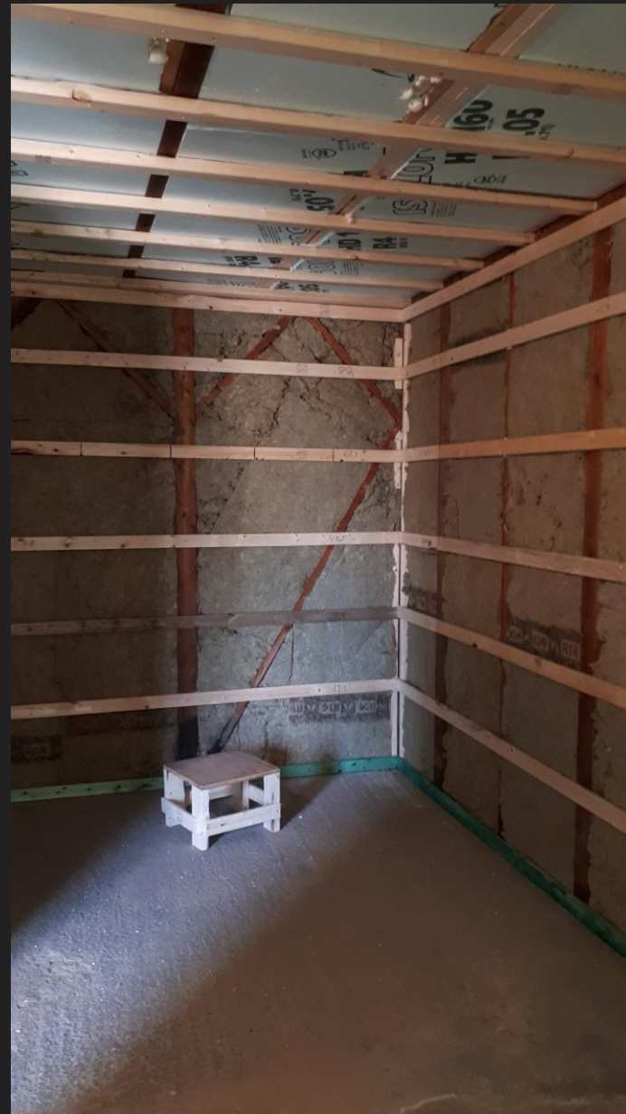
From Left: New wall creating Propagation Room; Pictures of drop ceiling and wall insulation going in.
