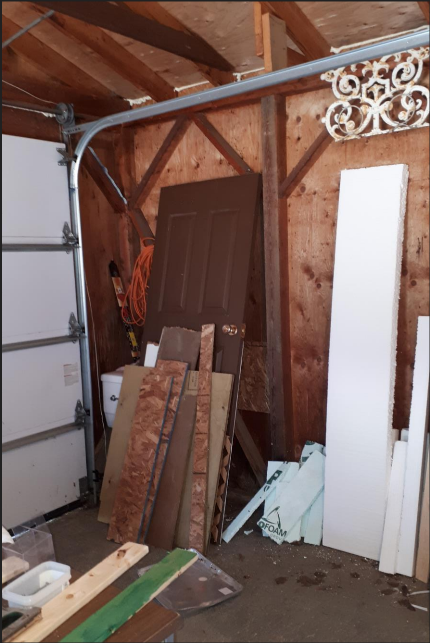
Garage SW Corner BEFORE
