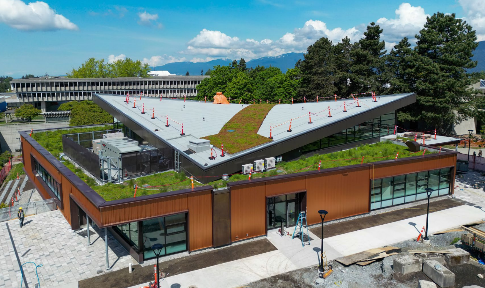
First Peoples' Gathering House under construction, May 2025
