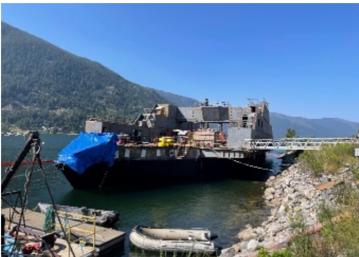
New vessel construction showing tunnel bridge installation well underway.
