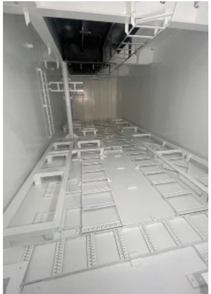
Photo of switchboard room fully painted on new vessel.
