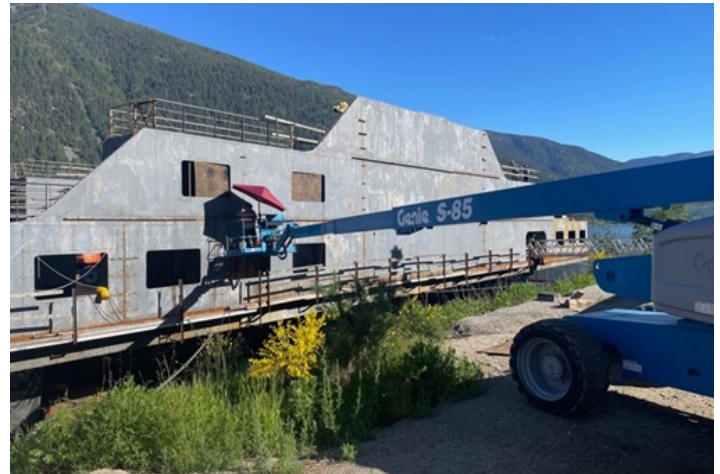
Photo of ongoing welding on external superstructure on new KLF vessel.
