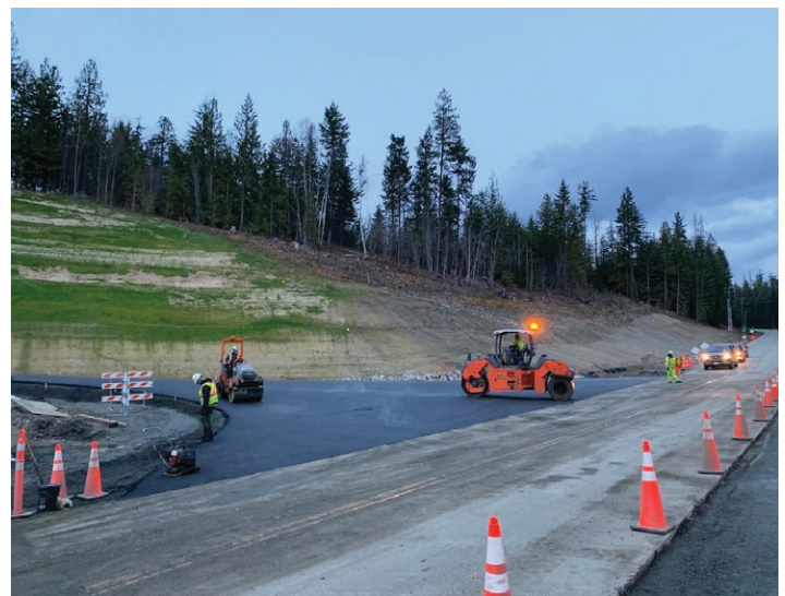
Paving the tie-in from Upper Balfour Road to Highway 3A.
