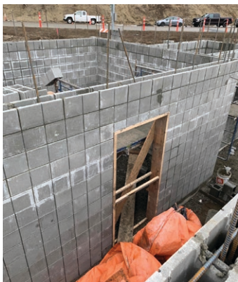
The Balfour terminal washrooms are nearing completion.
