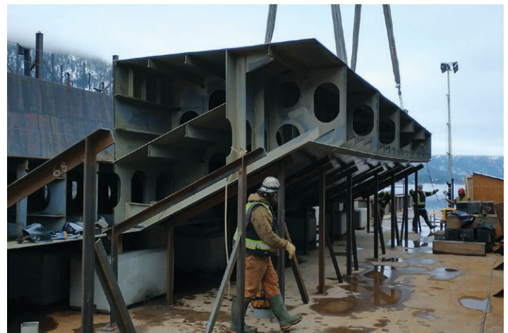
Engine room blocks are assembled in the drydock.
