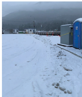
Stockpiled snow against the bus pad at Balfour.
