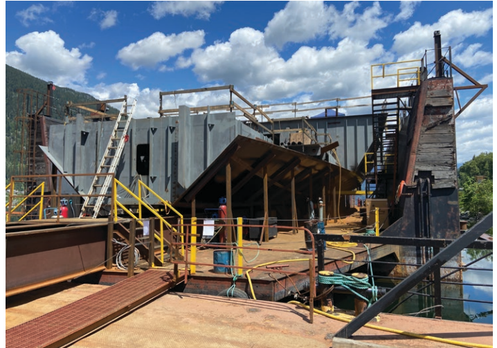
Vessel hull assembly on the drydock.
