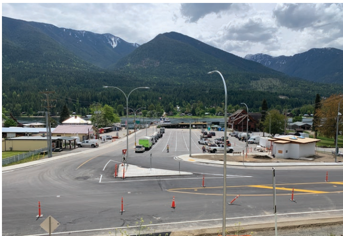
The repaved and newly upgraded Balfour terminal.
