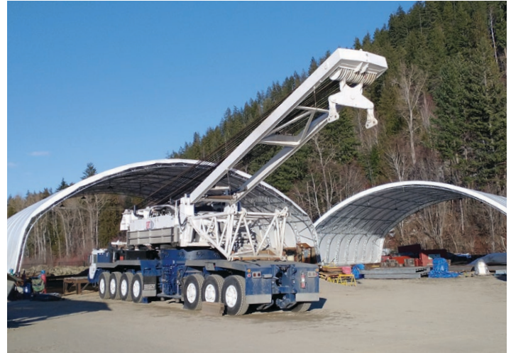
The new crane arriving on site at the end of February.
