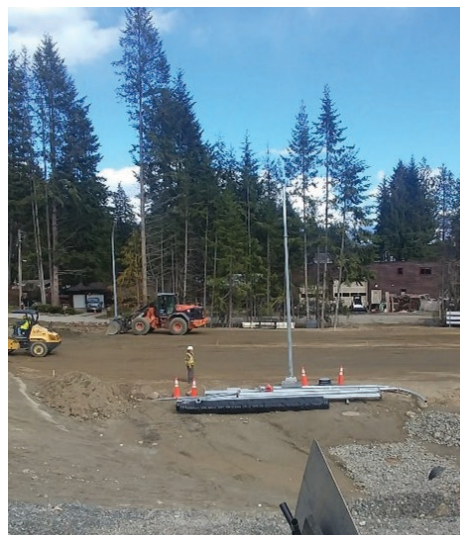
The new parking lot at Busk Road is nearing completion.
