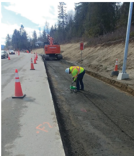
Repaving work is nearing completion on Hwy 3A/31.
