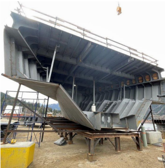
The bow section of the vessel on temporary supports ready for assembly to the main hull on the floating dry dock.
