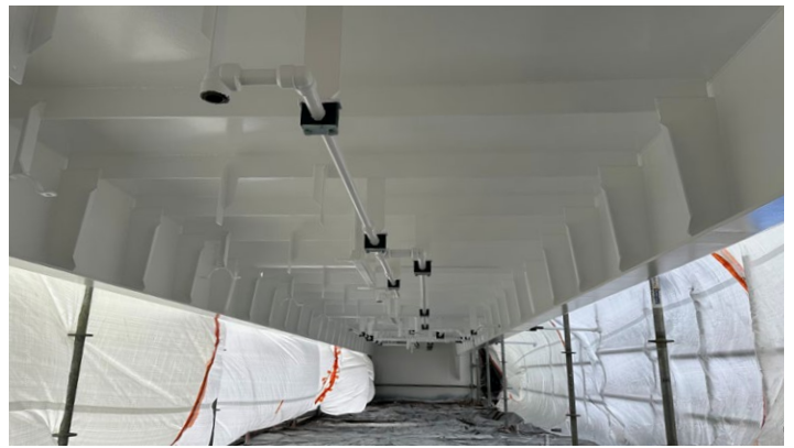
In the below tunnel, 100% of the preoutfit has been completed.
