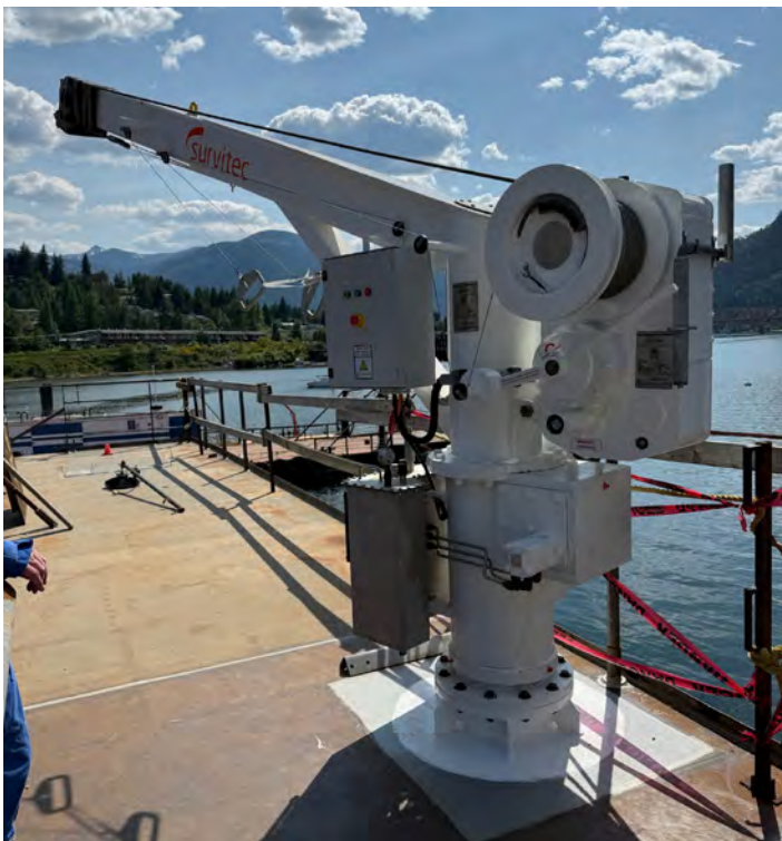
The rescue boat davit has been installed.
