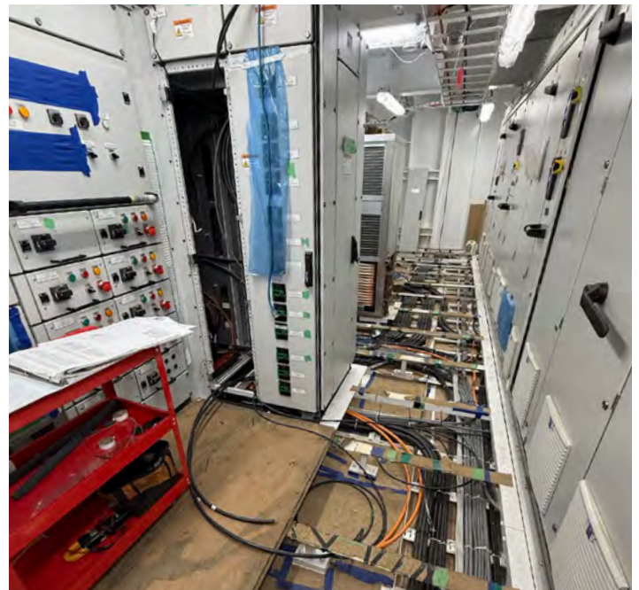
The switchboard room cabling being installed.
