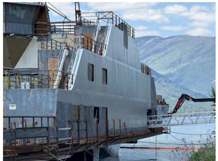
External painting of the new vessel's superstructure is under way.
